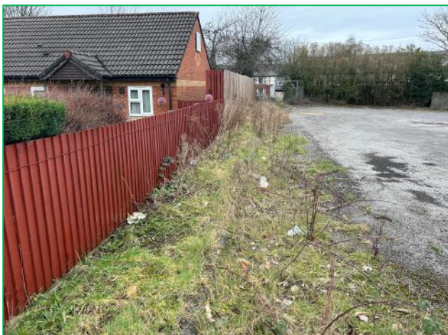
Looking north along the western boundary
