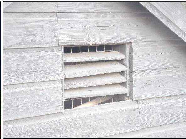
Figure 7: The louvred vent in the eastern gable end.
