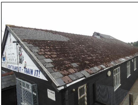
Figure 3: The roof of the building.
