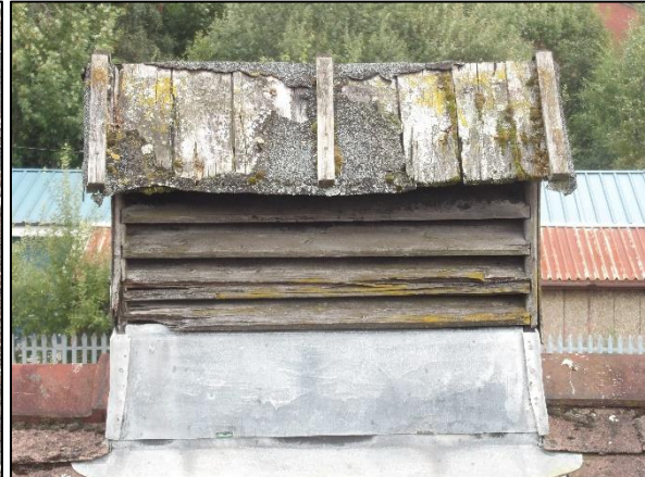
Figure 11: The vent structure.
