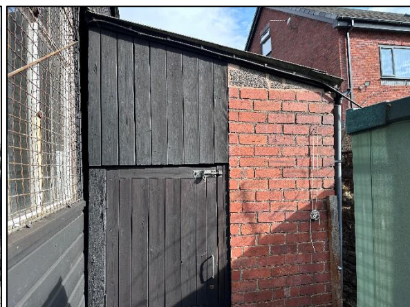
Figure 9: The lean to building to the east.
