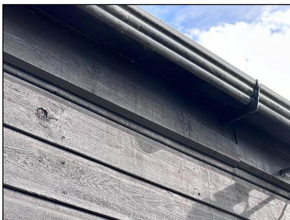
Figure 8: The tight-fitting fascia board.
