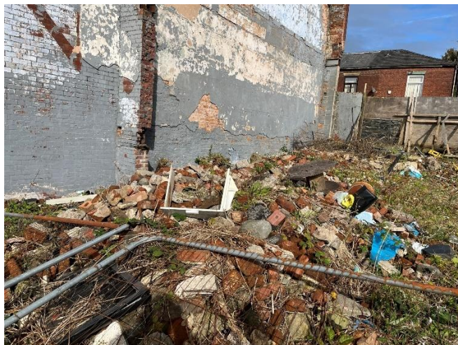
Photo 2: The brick and rubble piles on site.
