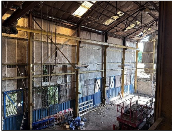
Figure 18: The interior of Area 2, viewed from Area 1.
