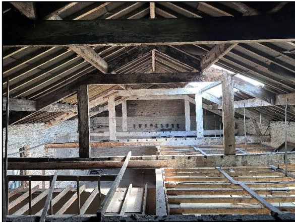
Figure 14: The roof structure in Area 1.
