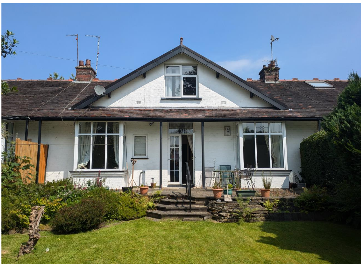
Fig 7. Images of the rear of 3 Broadhalgh Avenue
