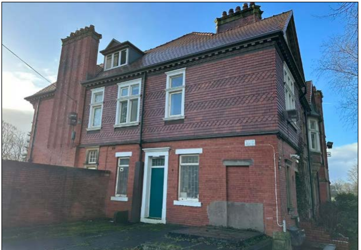
5. The east elevation has a plainer appearance
