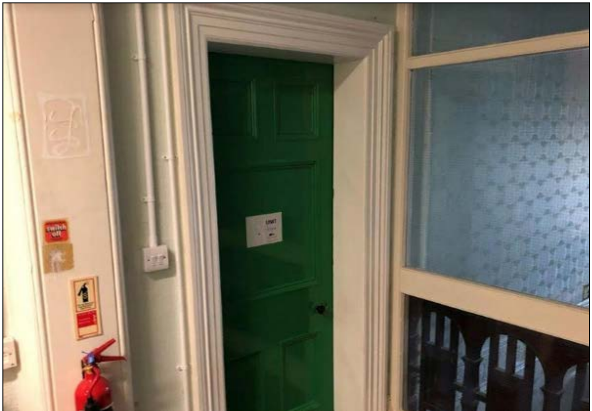
10. First floor panelled door and moulded architrave
