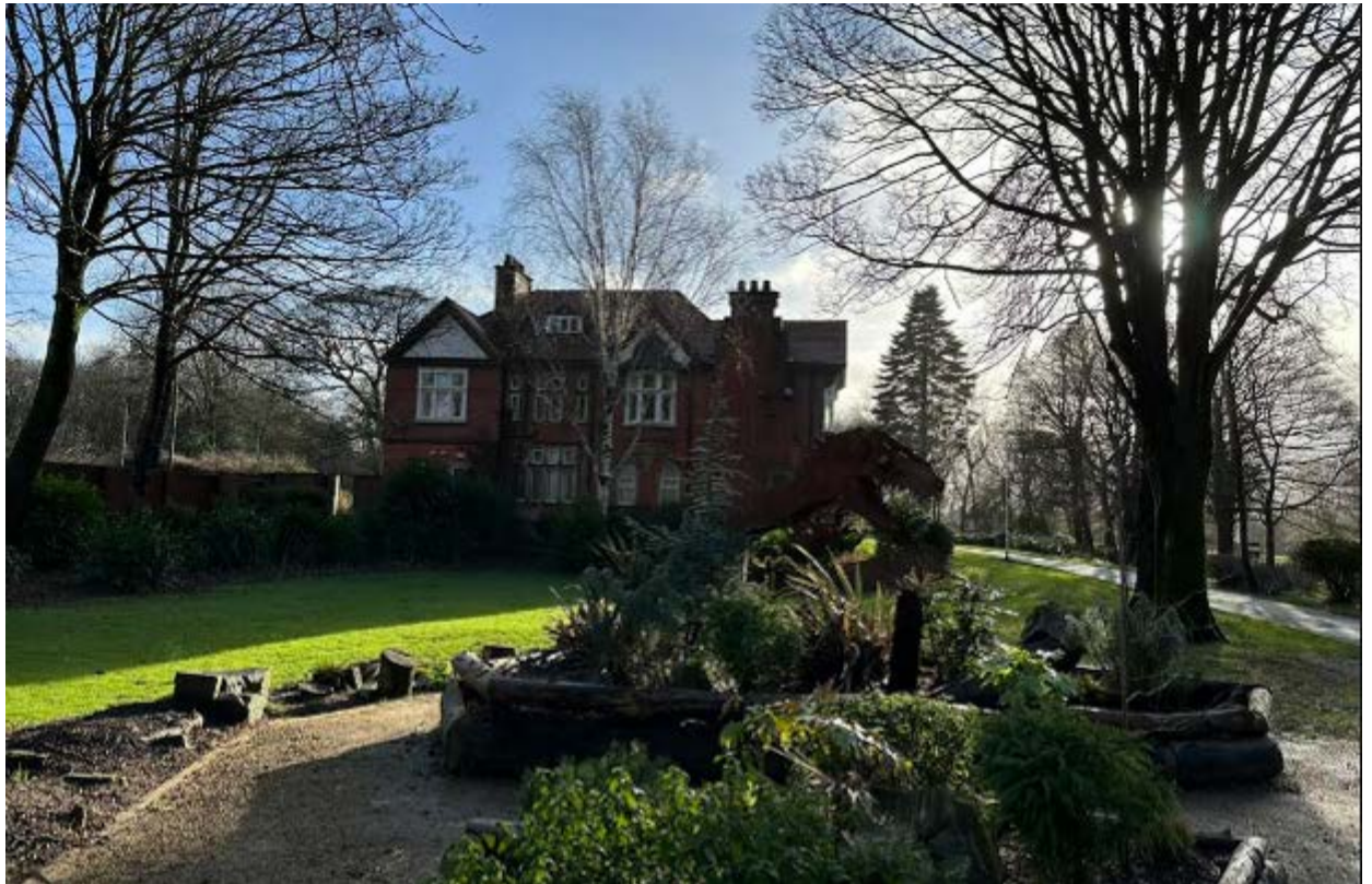
13. The building stands predominant in views throughout the park
