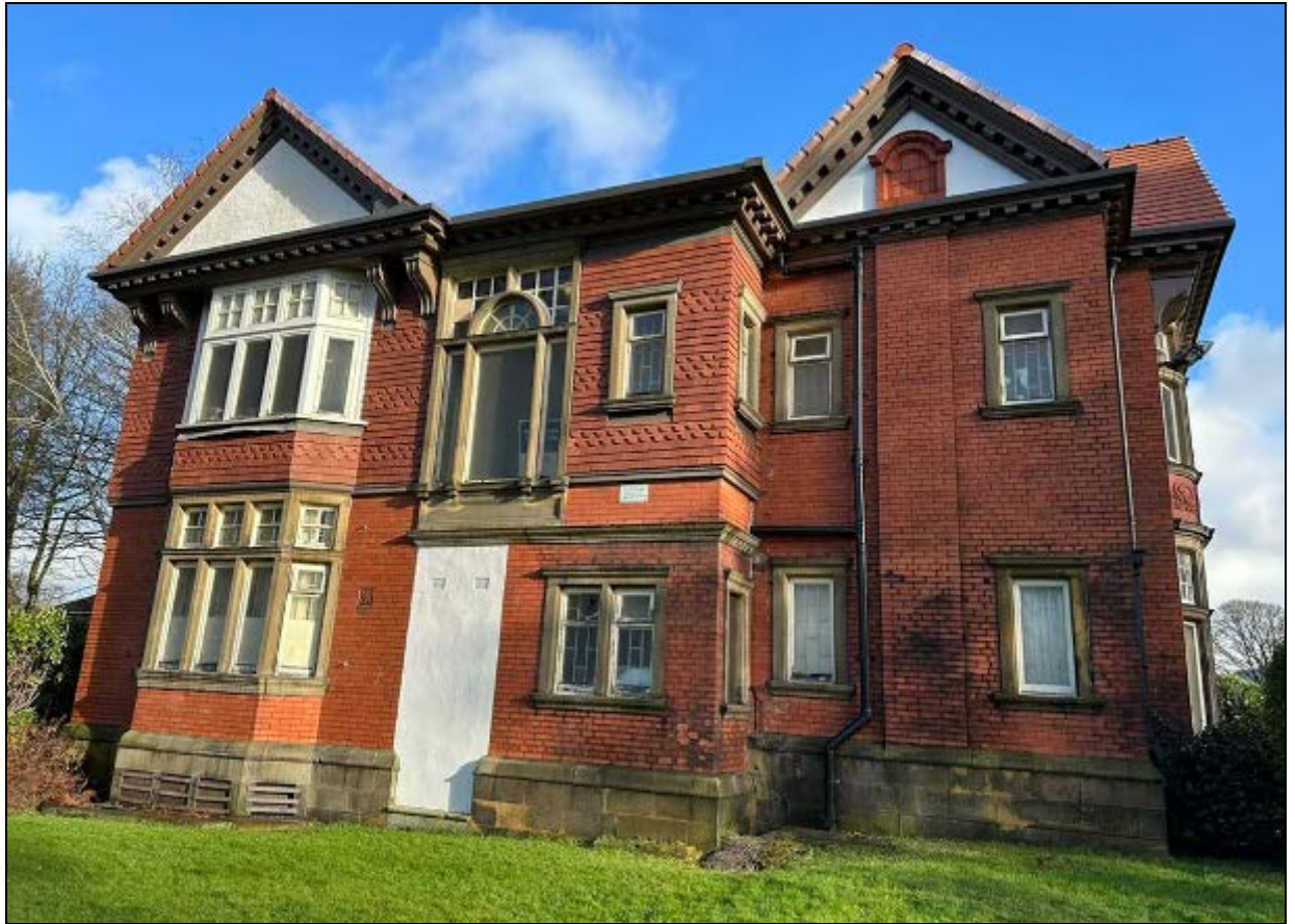
4. West elevation with tall stairlight and tile hanging
