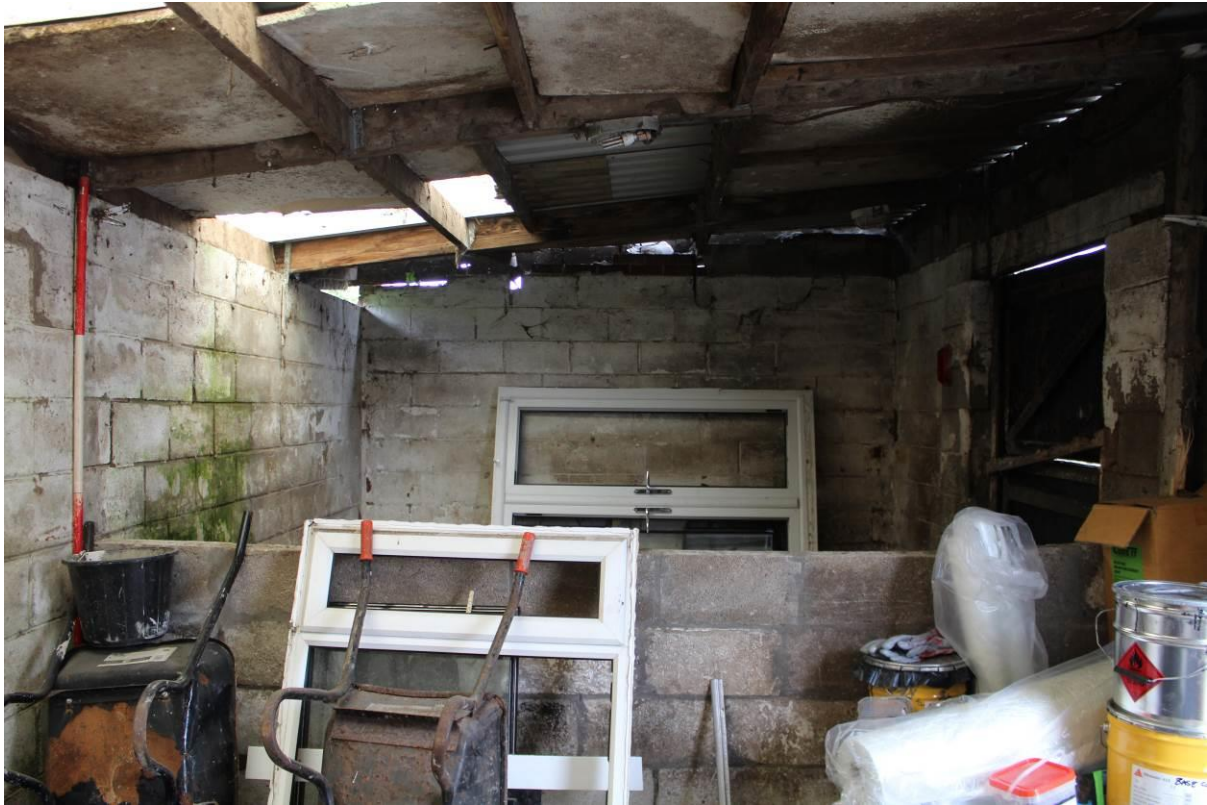
Photo 46: Interior of Stable Block B, looking SE
