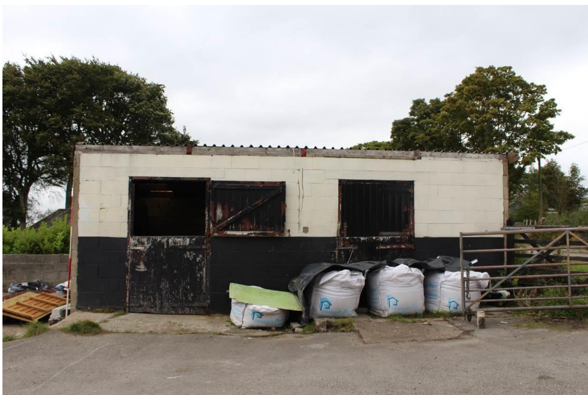
Photo 43: Front Elevation of Block B, looking NE
