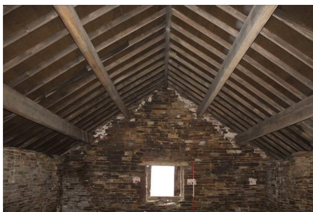
Photo 26: Interior of Barn B: General view of First Floor; showing roof detail, looking NW
