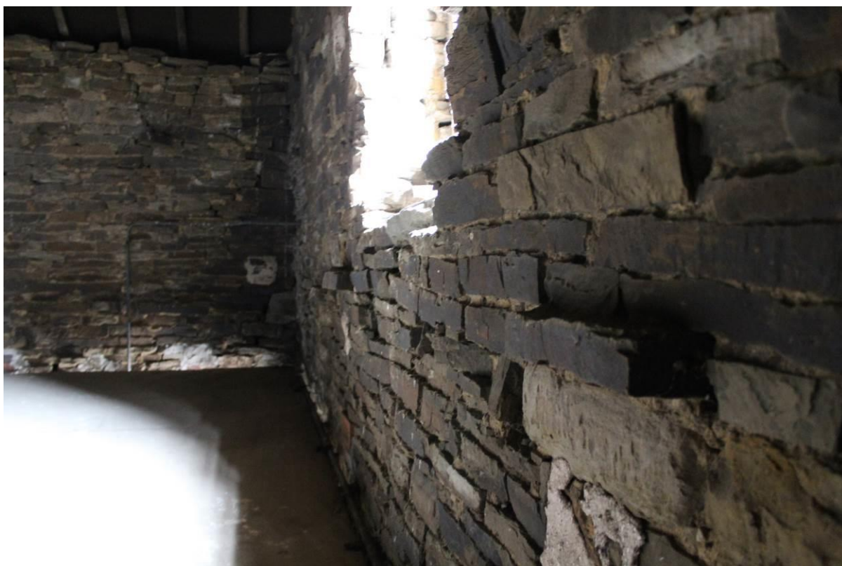
Photo 30: Interior of Barn B: General view of First Floor; showing window and protruding stone plinths detail, looking SW
