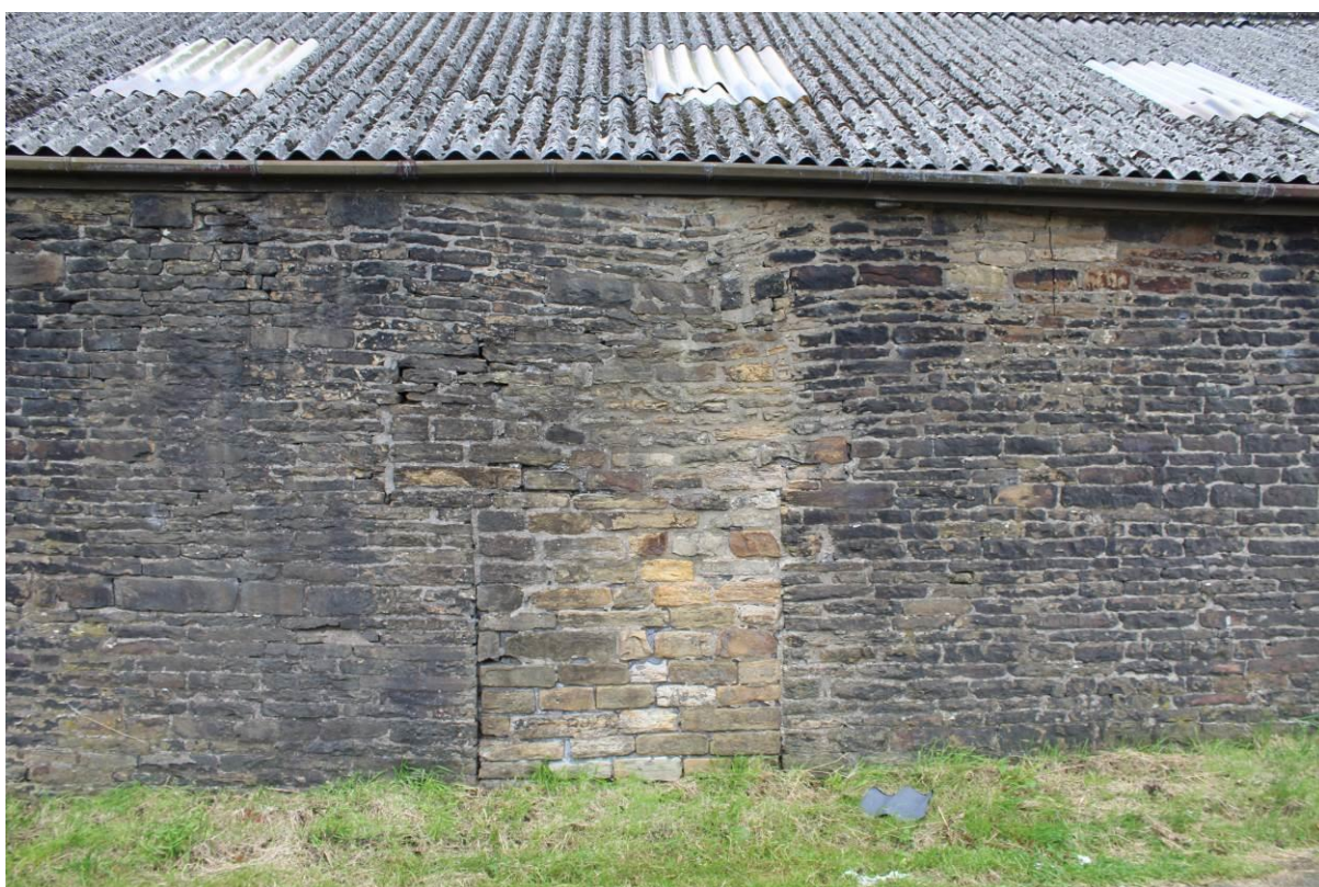
Photo 3: Front elevation of the Barn A, note blocked up doorway, looking NW
