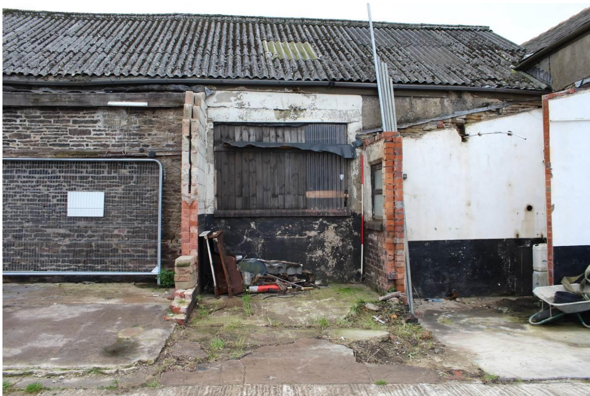
Photo 10: Rear elevation of Barn A; showing extensions partially demolished, looking SE
