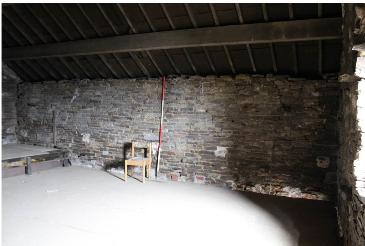
Photo 32: Interior of Barn B: General view of First Floor; showing blocked up beam slots, and protruding stone plinths, looking S
