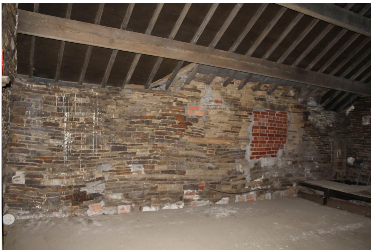
Photo 31: Interior of Barn B: General view of First Floor; showing blocked up window and undulating stone courses detail, looking E
