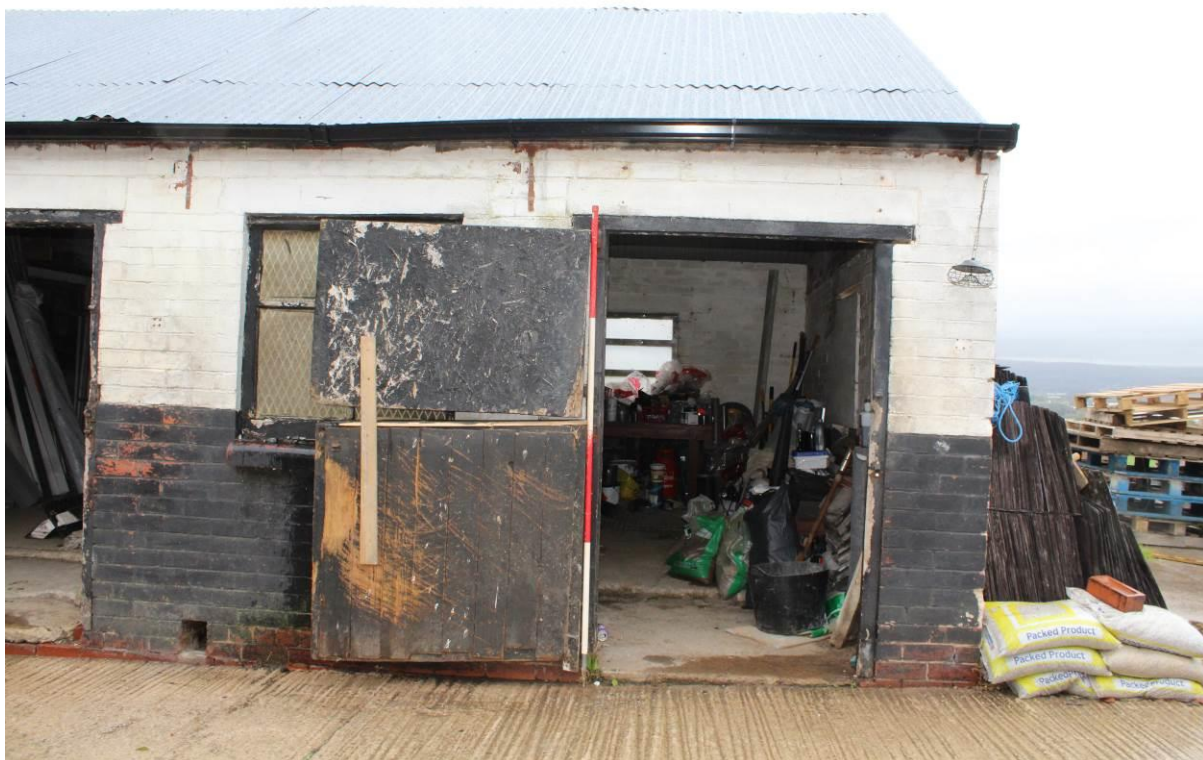
Photo 36: Front elevation of Stable Block A, looking NW
