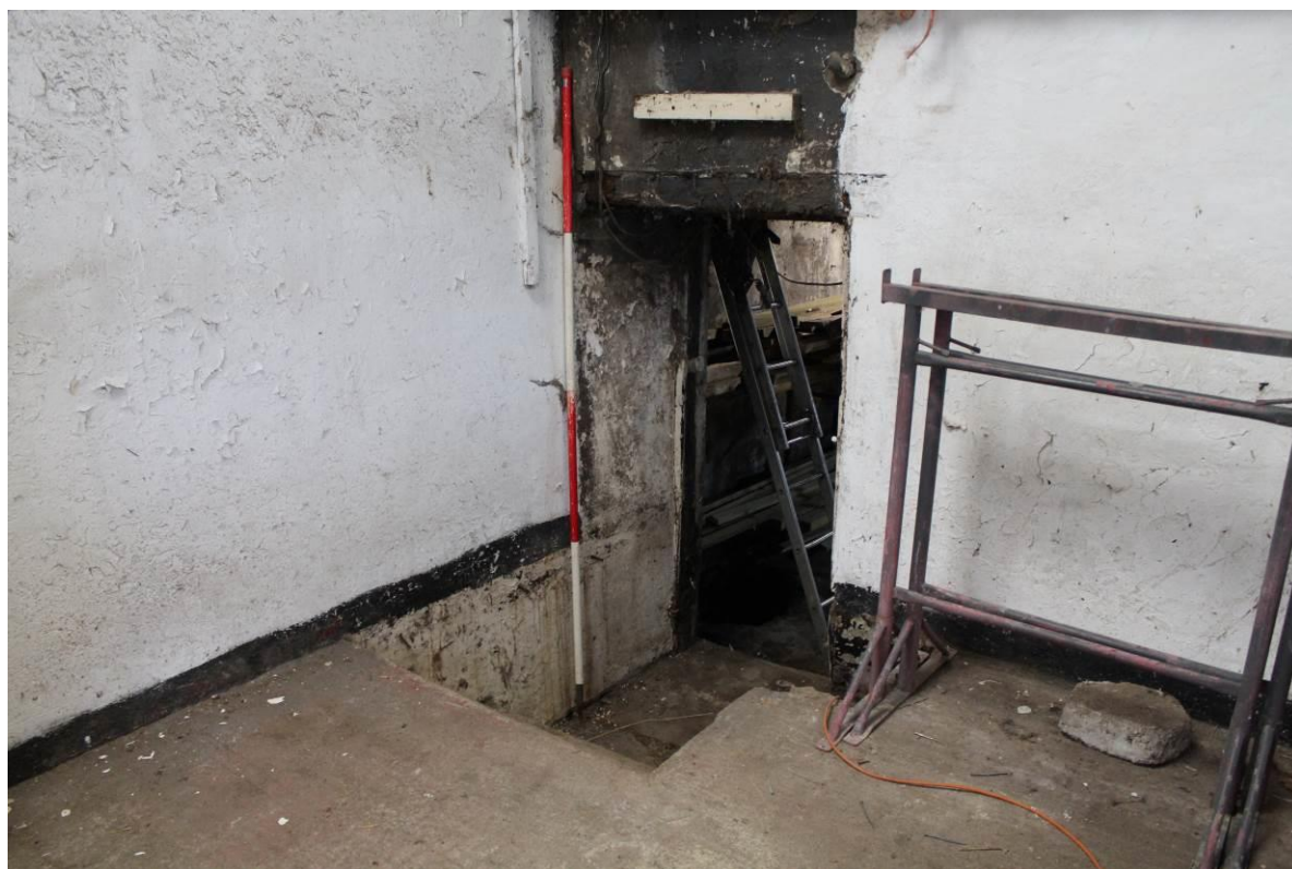
Photo 20: Interior of Barn A, looking toward Barn B, looking S
