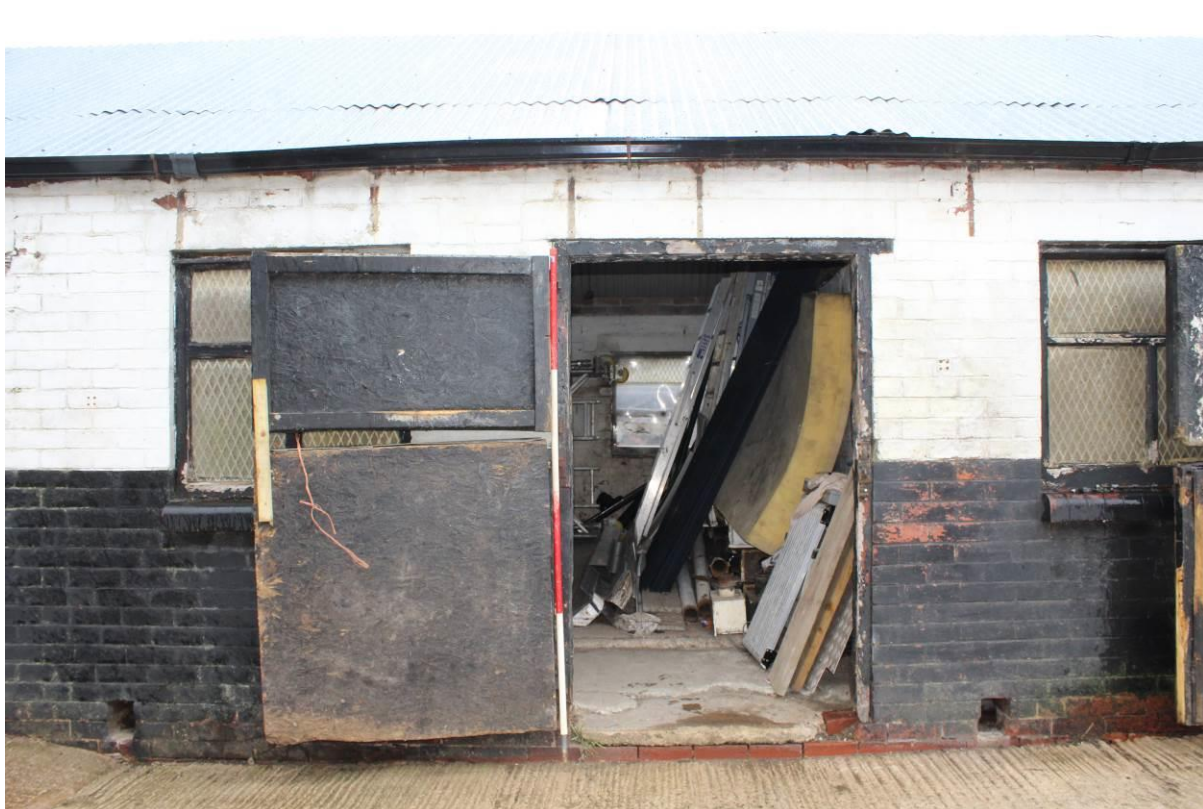
Photo 38: Front elevation of Stable Block A, looking NW
