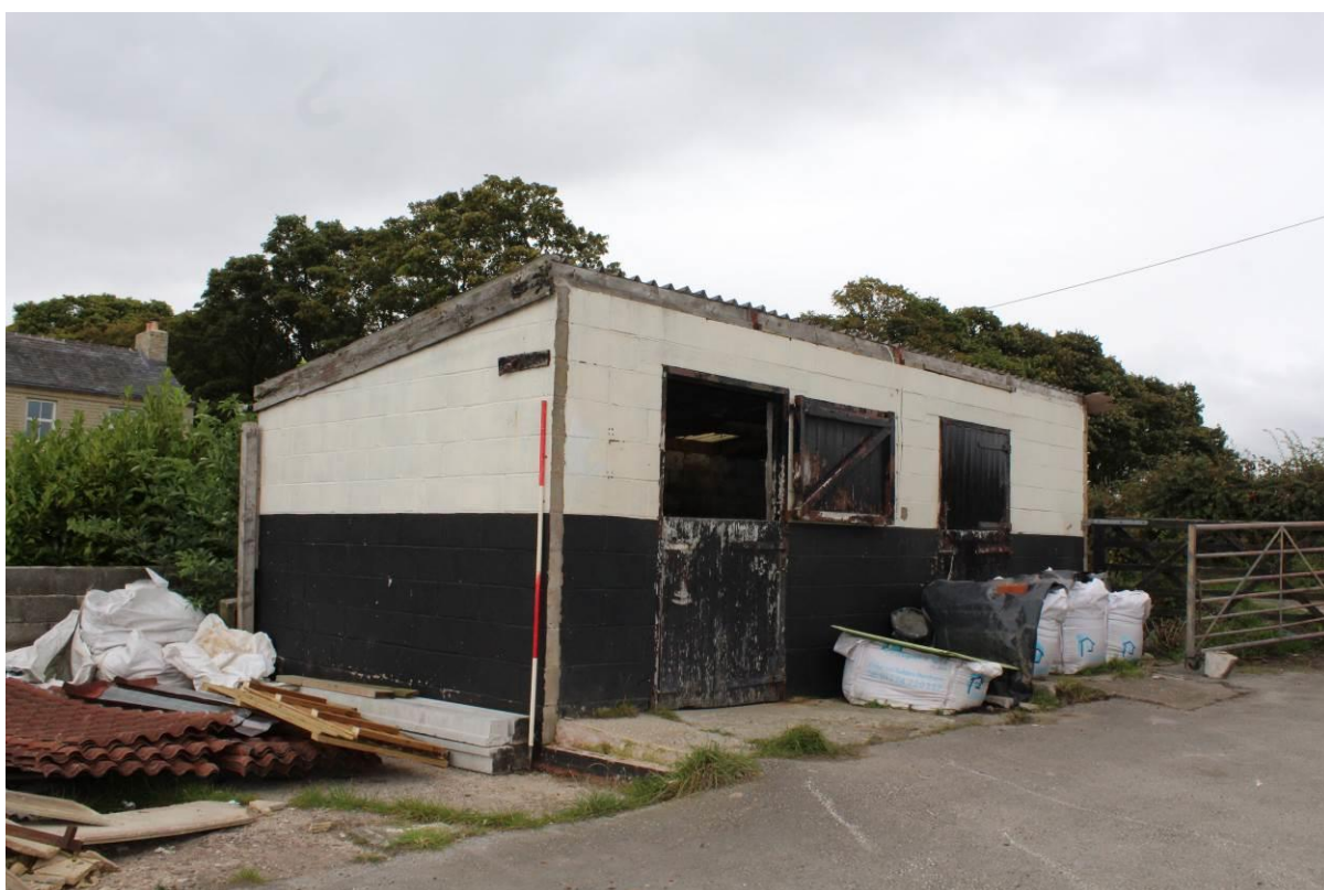
Photo 42: General View of Stable Block B; side and front elevation, looking E
