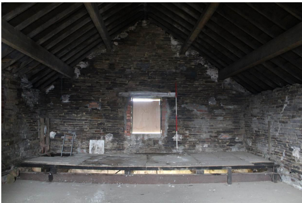
Photo 28: Interior of Barn B: General view of First Floor; showing window detail and elevated floor, looking SE
