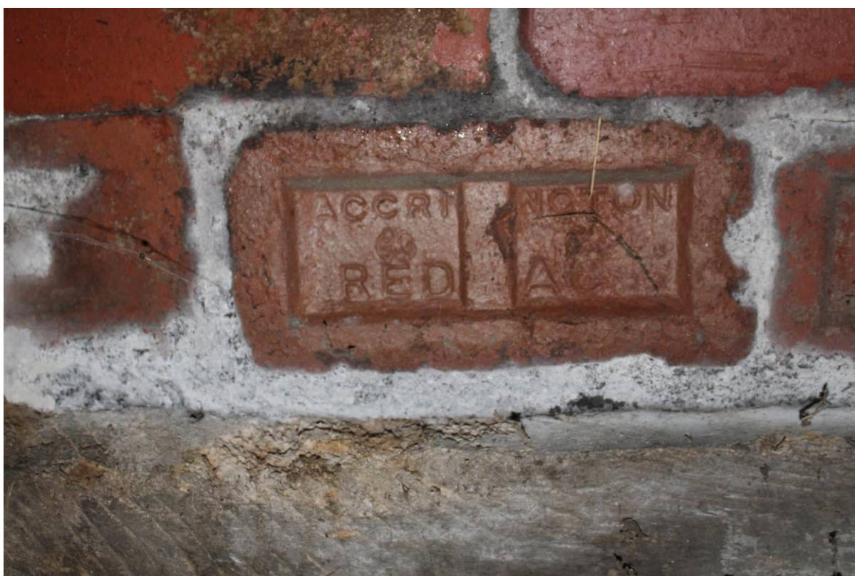
Photo 24: Interior of Barn B; blocked door detail with closeup of the upper course of bricks, looking NE (lower image inverted for clarity of inscription)
