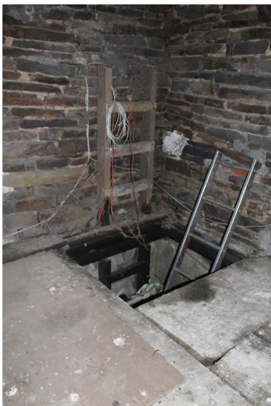
Photo 33: Interior of Barn B: General view of First Floor; showing access point; hatch and ladder, looking E
