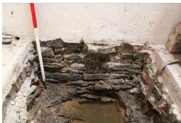
Photo 17: Interior of Barn A, Test pit in the SE corner, detailing packing, floor layers and foundations, looking NE and SE
