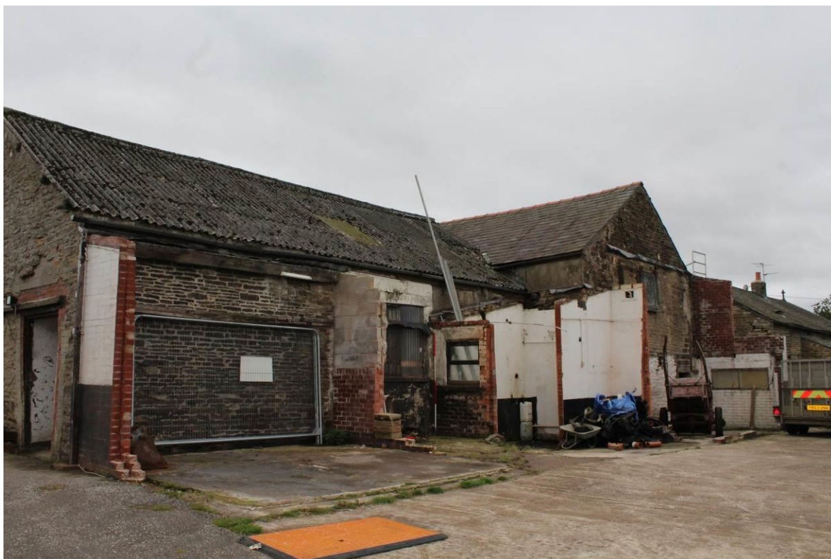
Photo 8: Side and rear elevation of Barn A and B, looking south
