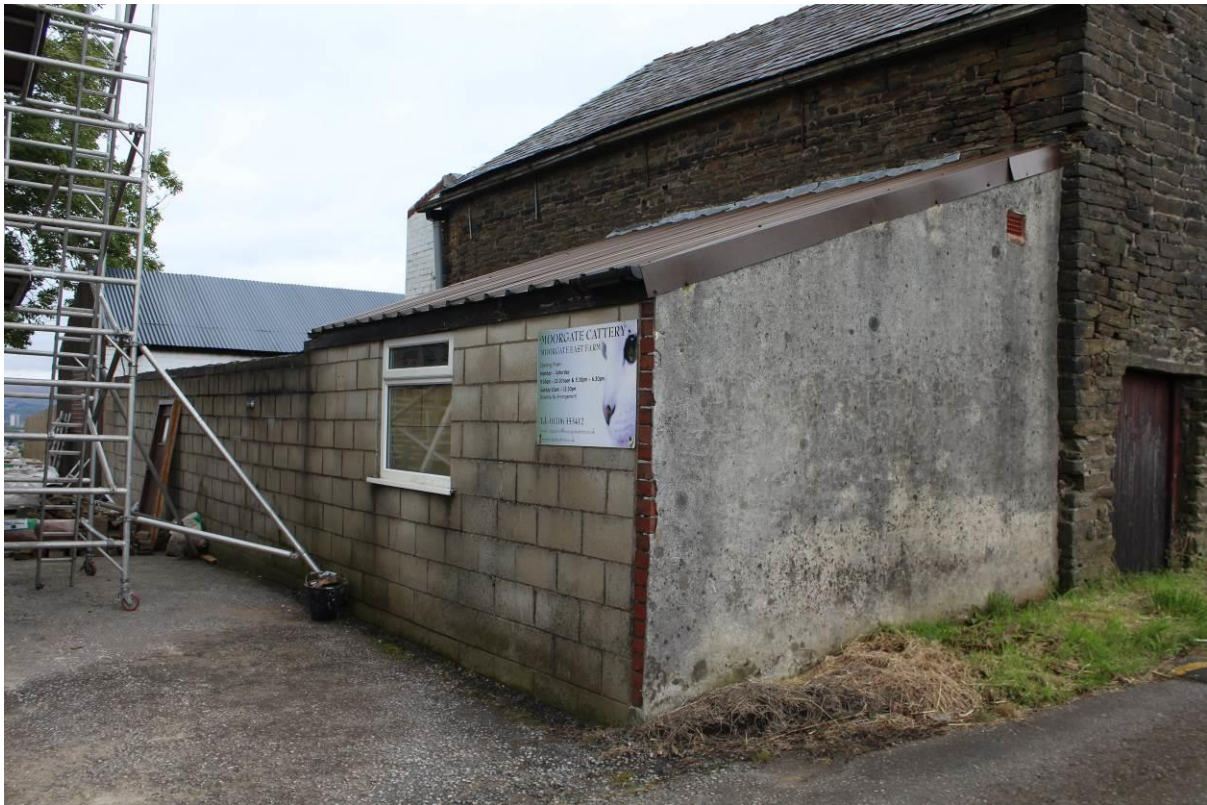
Photo 6: Front and side elevation of Barn B, and a 20 th Century lean-to, looking N
