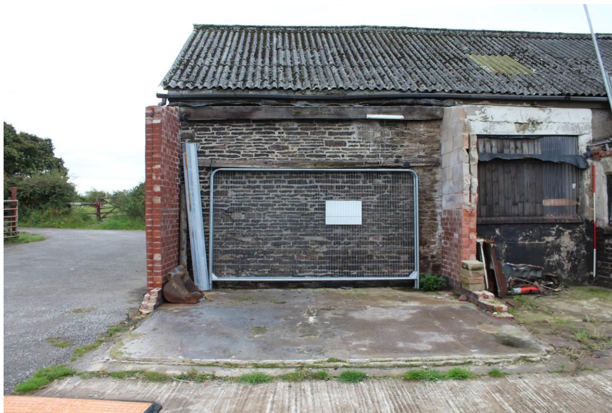
Photo 9: Rear elevation of Barn A; showing extensions partially demolished, looking SE
