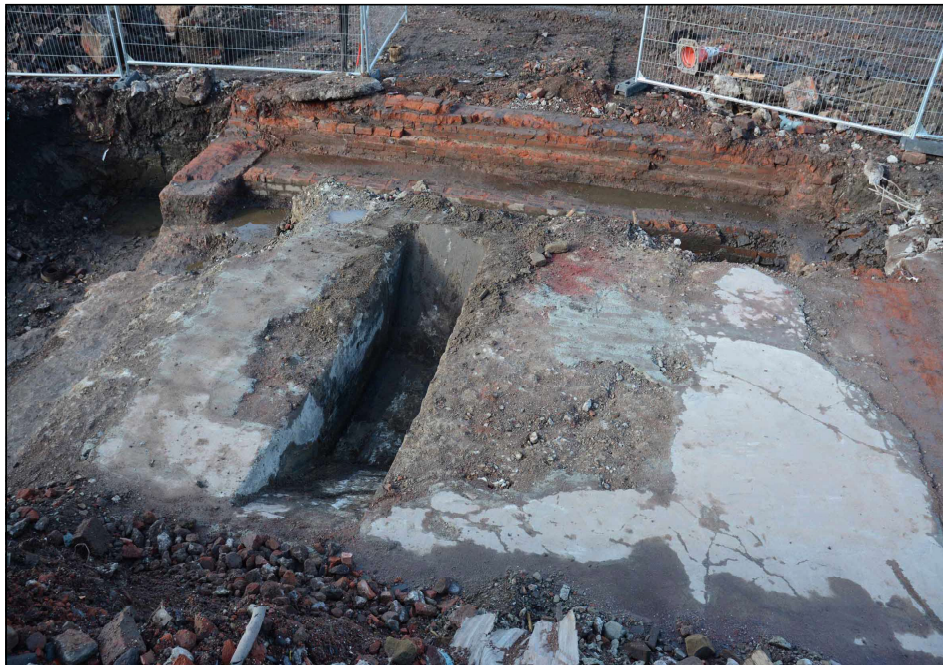
Plate 16. Trench 2, general photo, looking south
