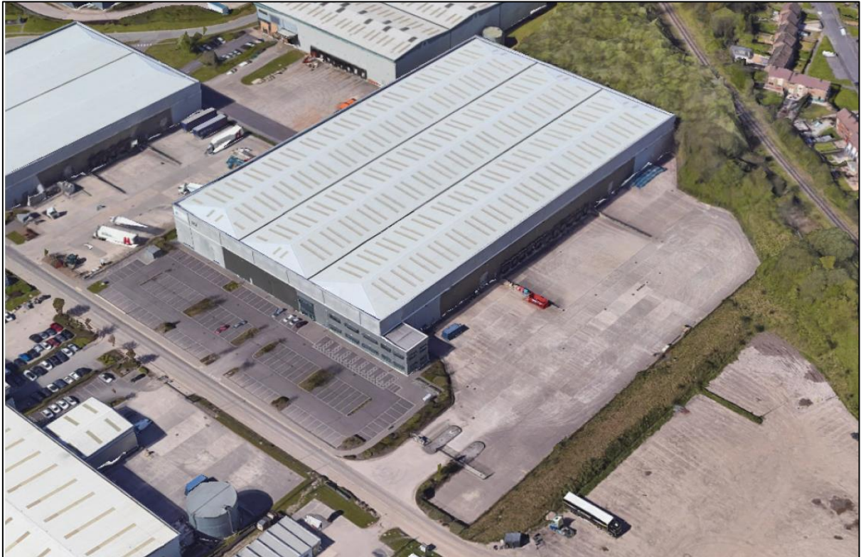
Figure 2: Existing access and warehouse at the Site
