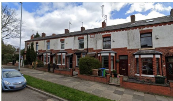
GP1 - Terraced properties at southern end of Heywood Old Road
