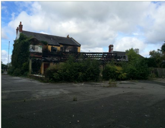
SP2 - Fire damage is evident to the rear of the property.
