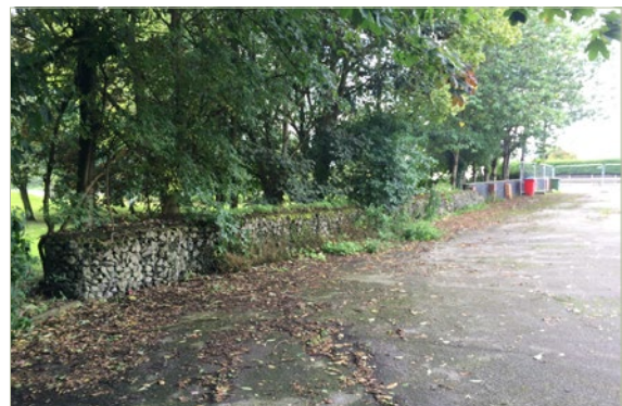
SP5 - Part gabion, part brick retaining wall along the southern boundary. Bitmac right up to the wall.
