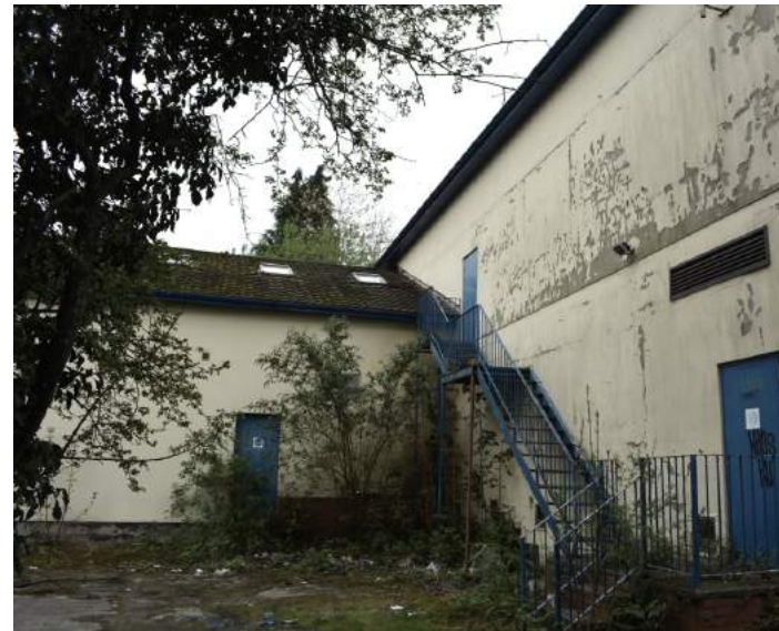
The main roof section to the right / the lower roof section to the left
