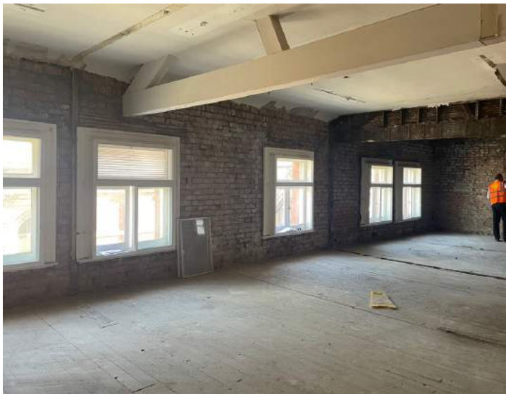
Interior After Strip Out
