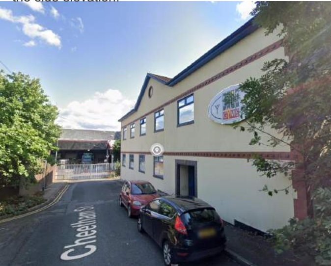
Front Elevation showing existing building materials
