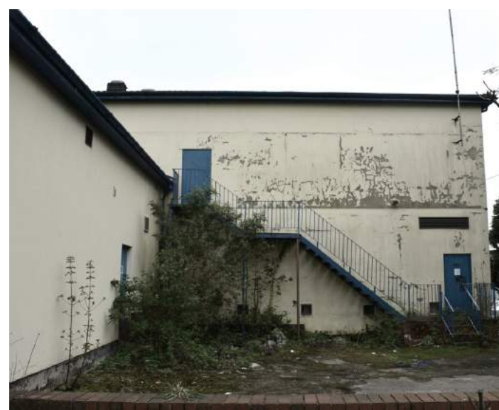
External Space to the rear of the building
