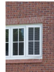
Window heads & sill detail
