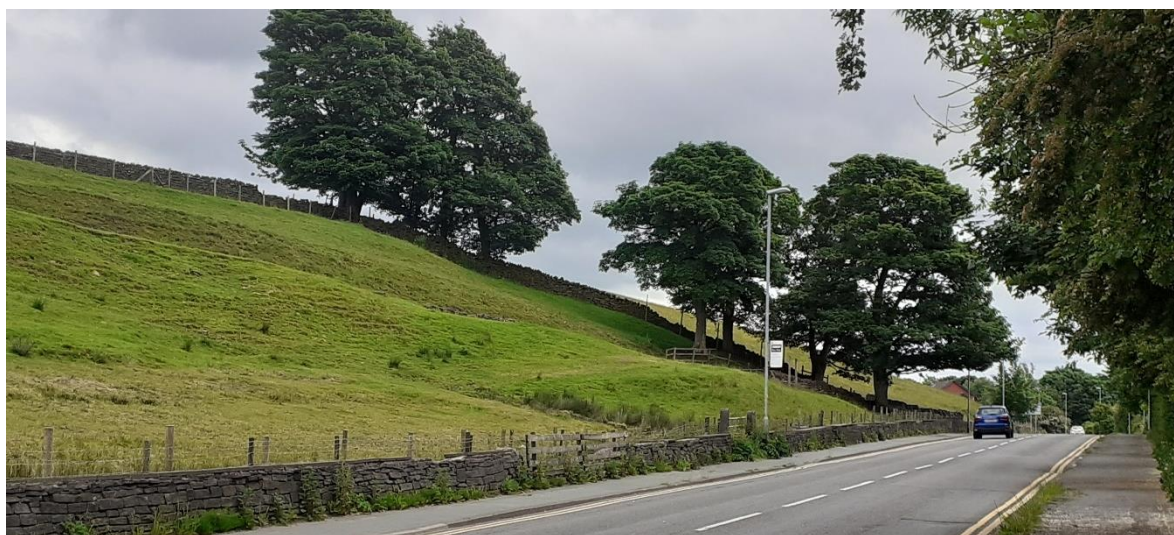
Figure 3- Photograph of site from north
