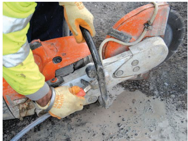
Figure 3 Water suppression on a cut-off saw
