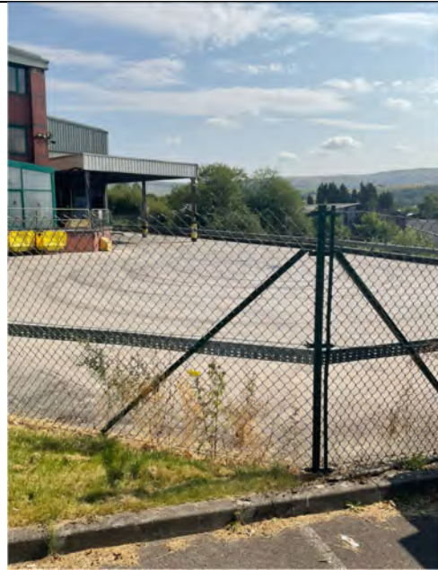
Carpark replaced with silos slab & foundations
