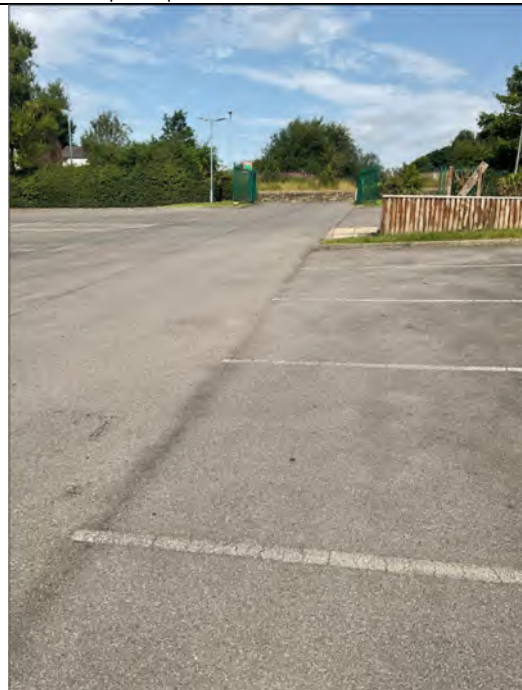
Site entrance to car-park
