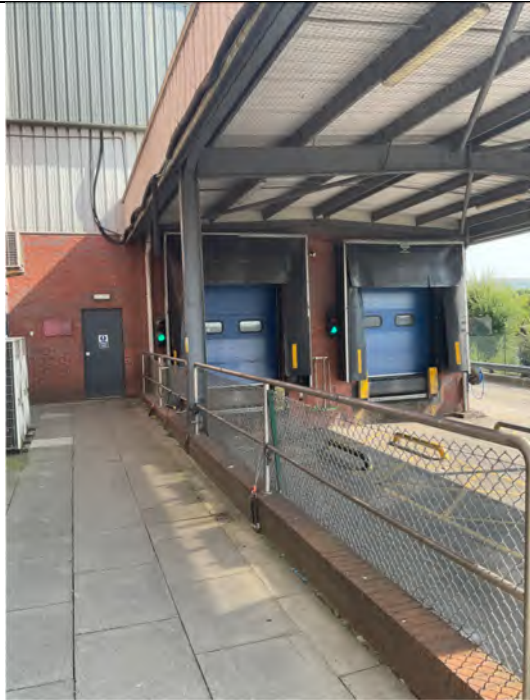
HGV loading bays
