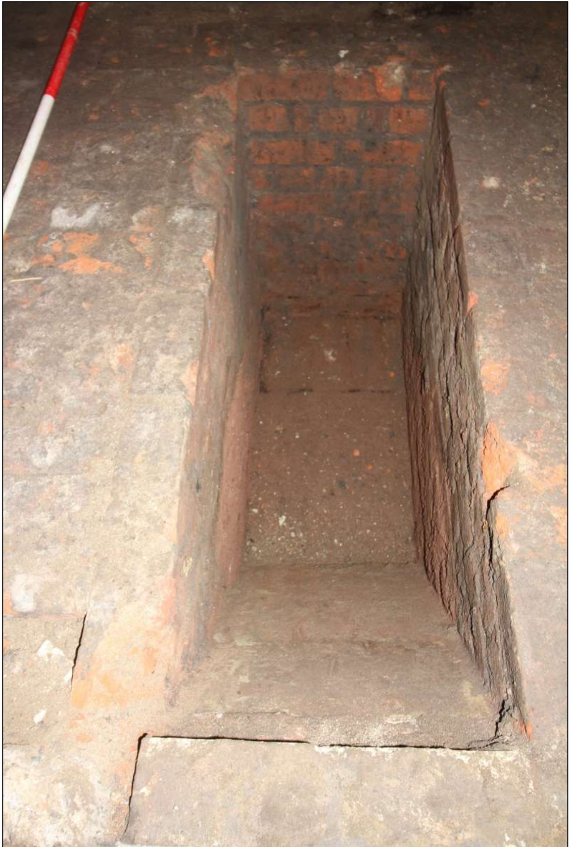
Plate 17: Detail of the brick structure below the floor of Room B119
