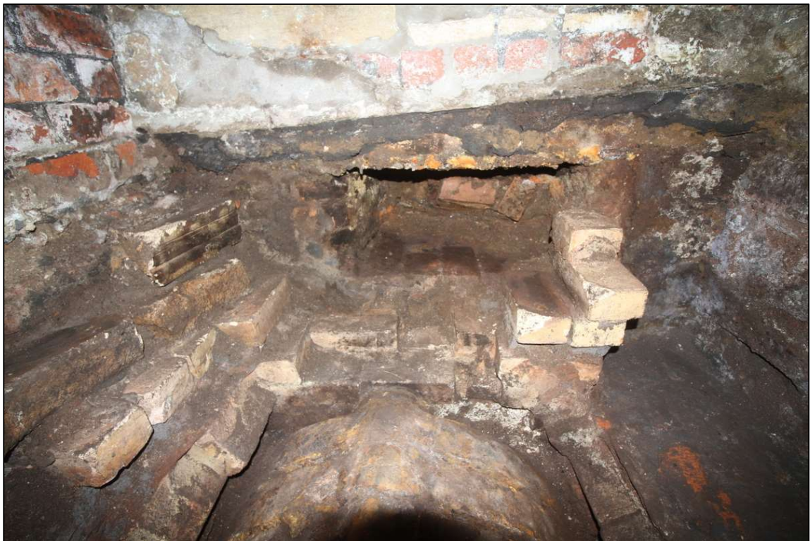
Plate 13: Detail of the rear flue to the saddle boiler
