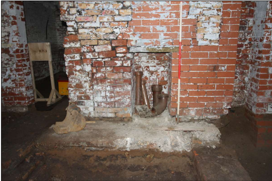
Plate 15: The fireplace within the southern wall of Room B120
