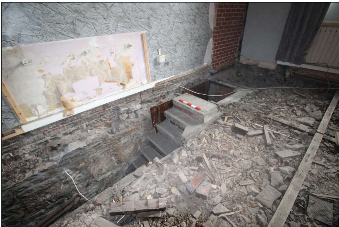
Plate 8: The upper section of the staircase below the removed floor within Room G6
