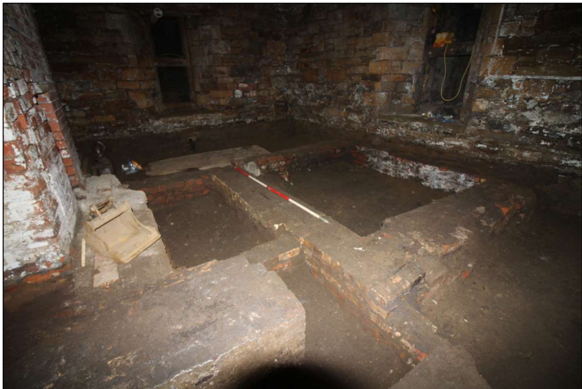
Plate 14: The brick walls discovered below the floor of Room B120
