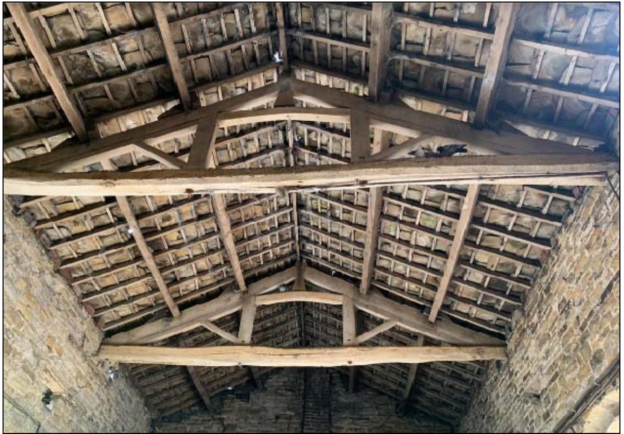
6. Kingpost trusses machine-cut, but with reused tiebeams
