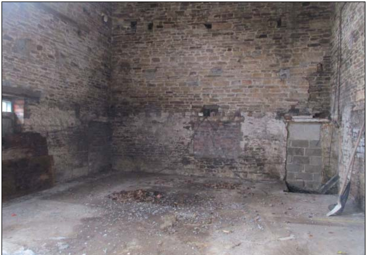
7. The third bay of the barn is open, but hayloft door indicates a floor once existed
