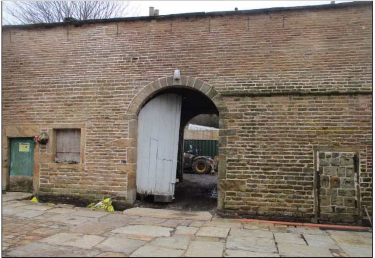
1. The barn at Lower Town House Farm: front elevation
