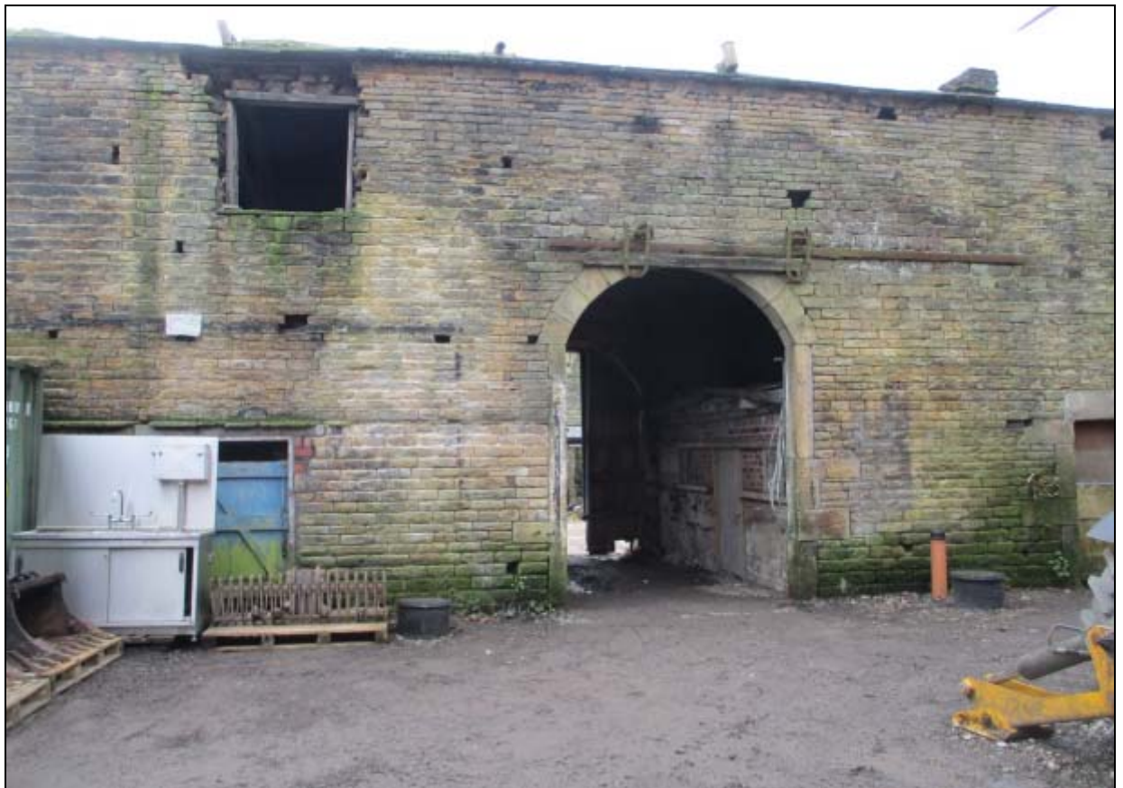
2. The barn viewed from the rear
