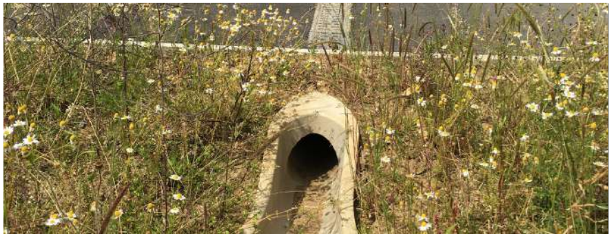
Precedent image of a rain garden
