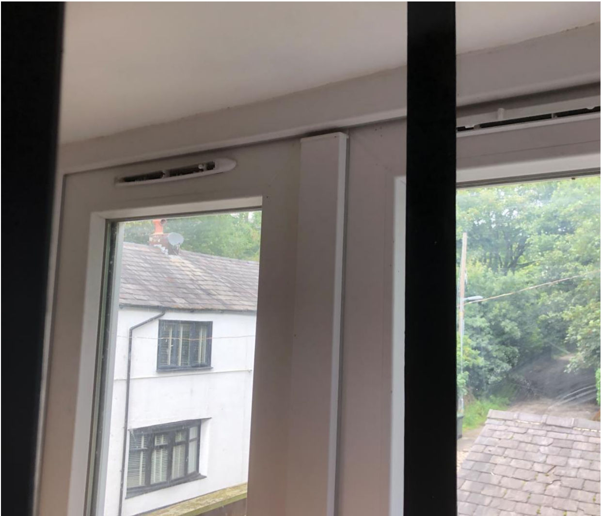
Figure 3: Picture Showing Open Trickle Vents
