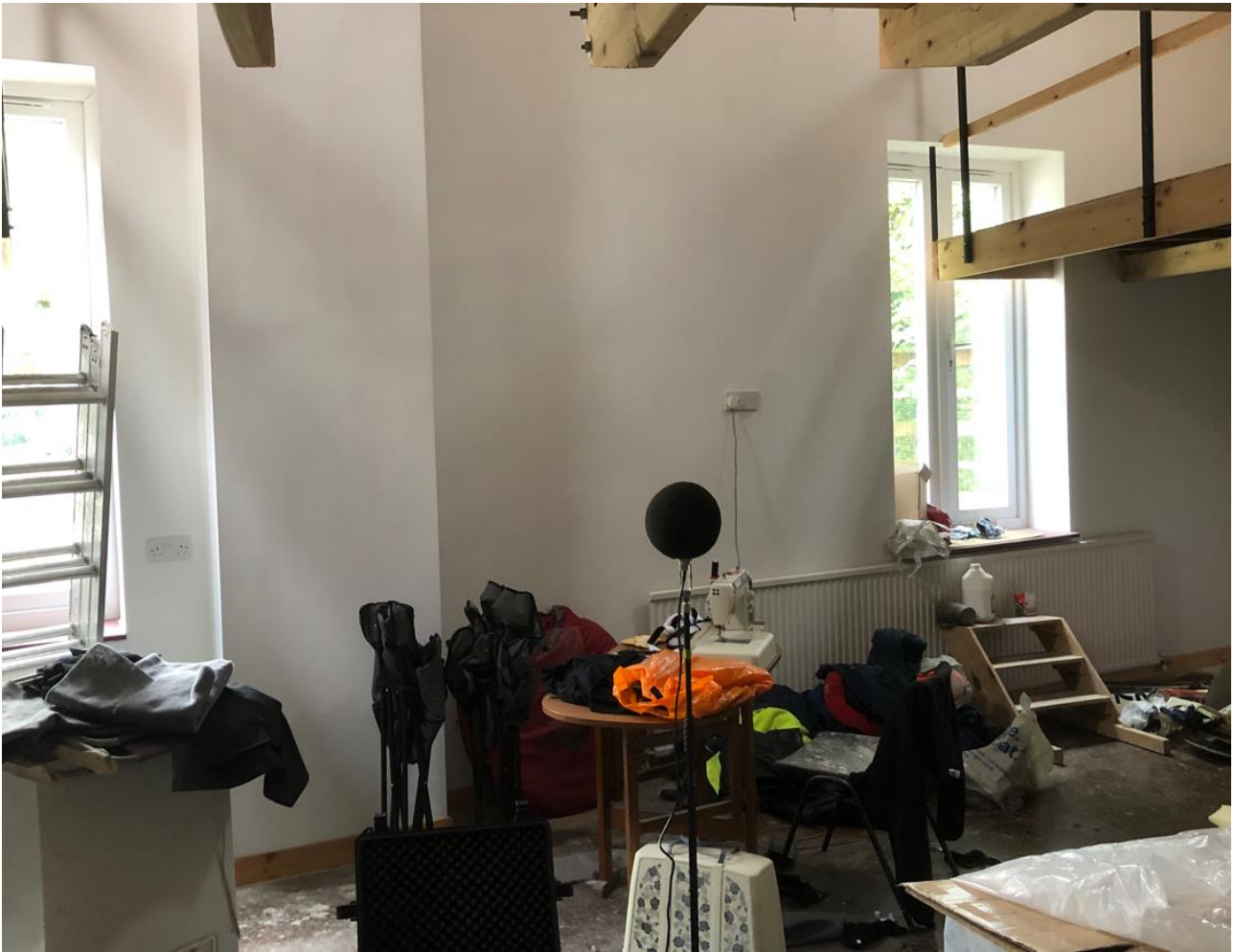
Figure 2: Picture Showing Monitoring Position 2
