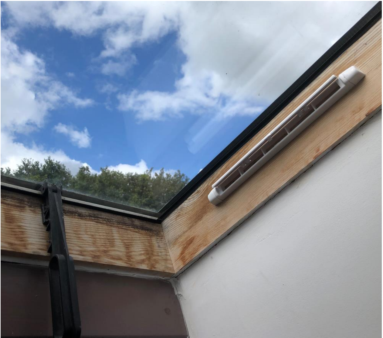
Figure 3: Picture Showing Skylight
