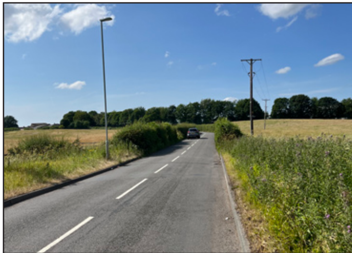
Context view (right) View on Whittle Lane from photo location
