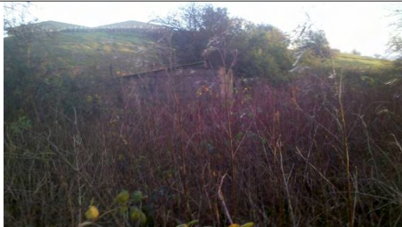
Northwest corner of site. Derelict building present in overgrown enclosure.
