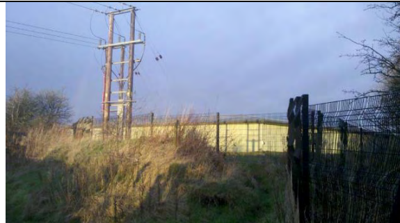
Large building forming part of adjacent industrial estate to the north of Cripple Gate Lane near northeast corner of site. 2 overhead electricity lines enter site from the north.
