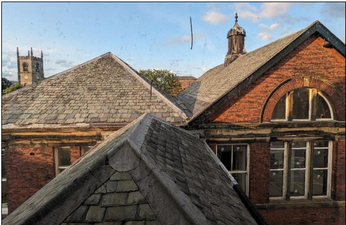
Plate 7. Looking northeast across roofs of Building Section 4 (in foreground) and Building Sections 1 (rear left) and 3 (rear right)
