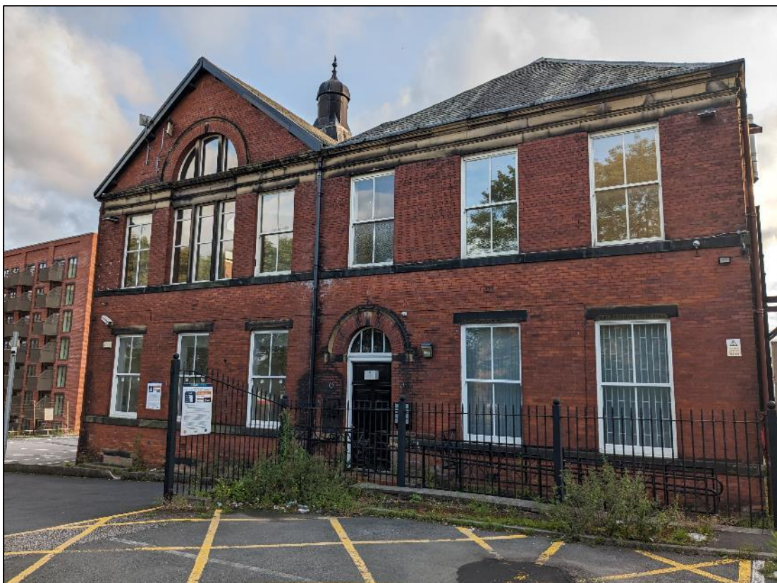
Plate 1. Northeast elevation of building, with Building Section 1 on right of image (hipped roof) and Building Section 3 on left of image (gable)
