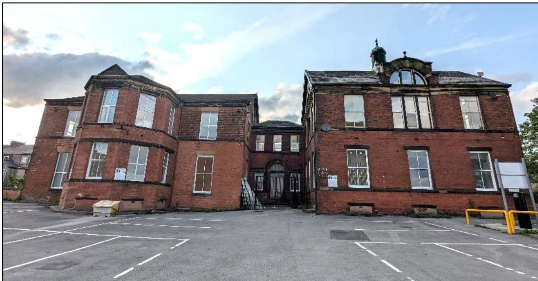
Plate 4. Building Section 2 on left of image, Building Section 4 (entrance) in centre, with Building Sections 3 on right of image
