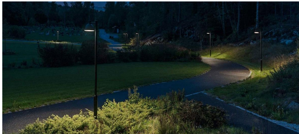
Column mounted lanterns illuminate pathways
