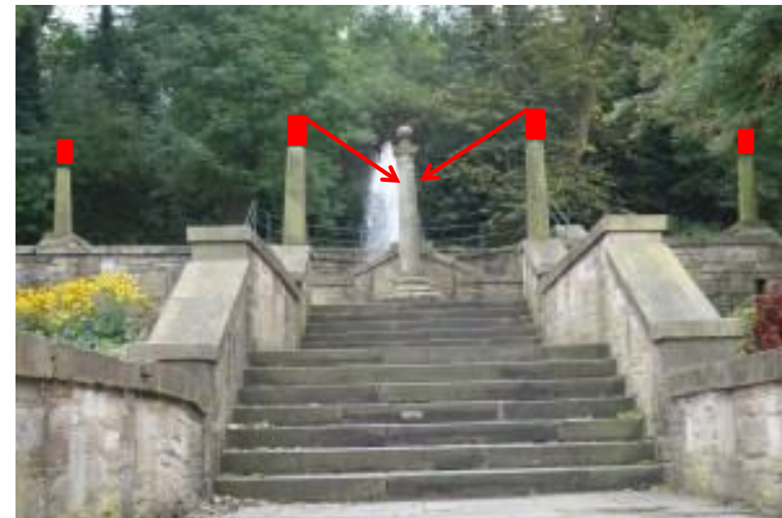
Condition of remaining stone obelisks and location of replacement lanterns. Spotlights to illuminate the Market Cross can be integrated within the new lanterns.
