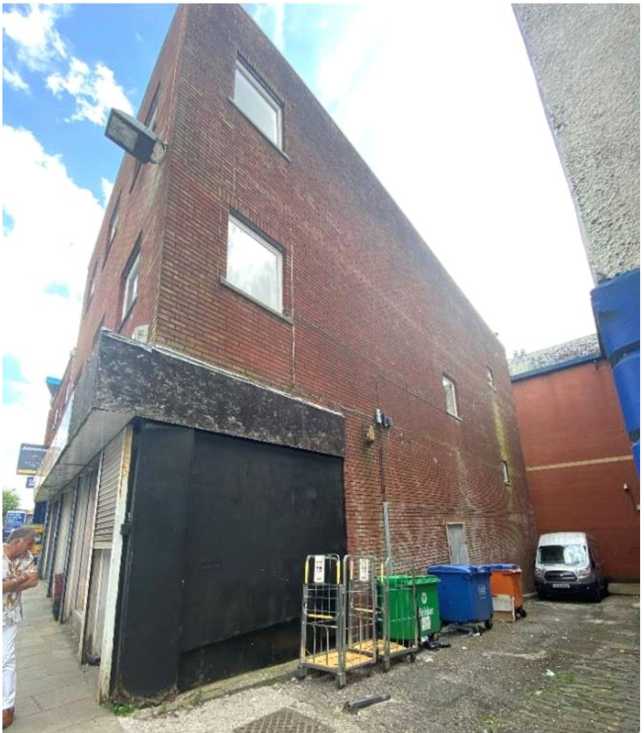
Photograph indicating current bins and loading area.
