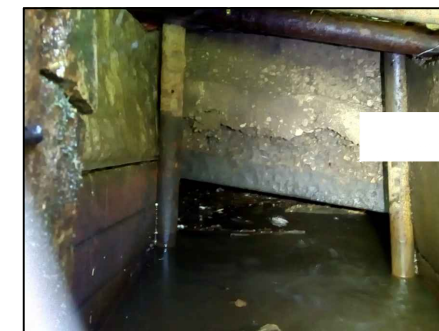
Photo 5: Beam partially blocking culvert under garage (Hopwood House)
