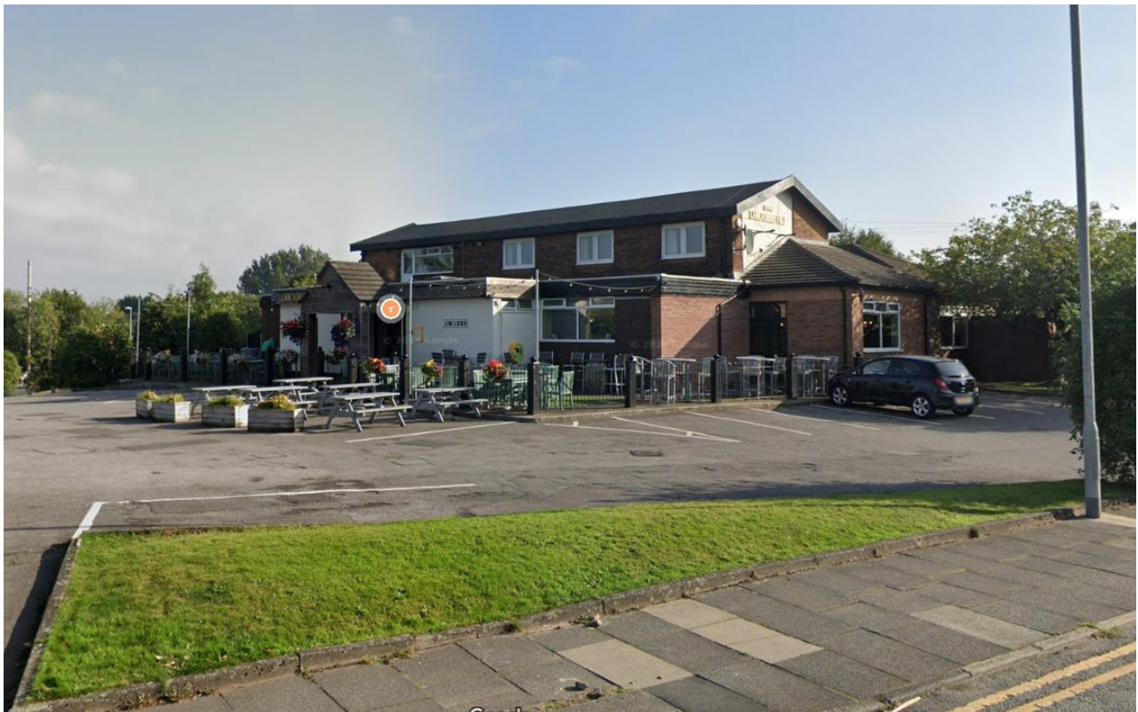
Image 3 - Photograph showing existing flat roof over existing single storey element fronting Kirkway and 3 car spaces in front of existing beer garden that have been used as an external seating area since 2020.
