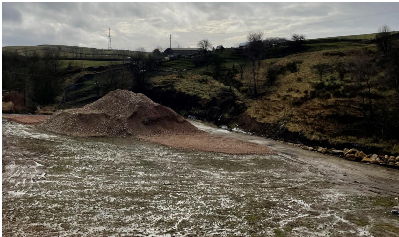
Demolition crush which has now been removed from Site.
