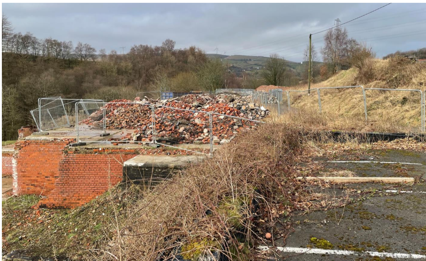
Demolition materials separated for removal.
