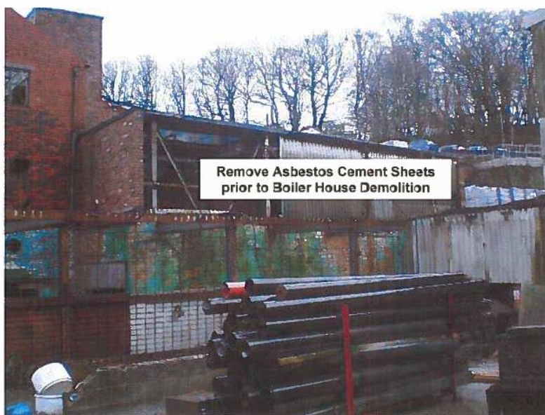
Asbestos Cement Sheets to be removed prior to Boiler House Demolition
