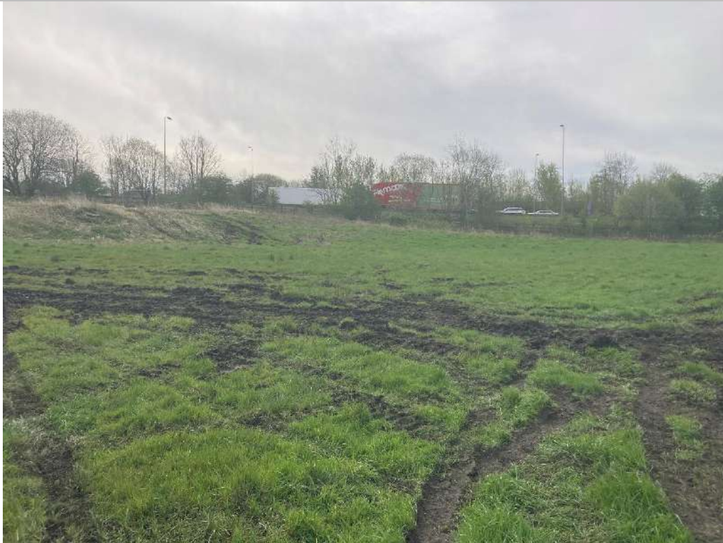
PLATE 5 SOUTH OF SITE POST WORKS
