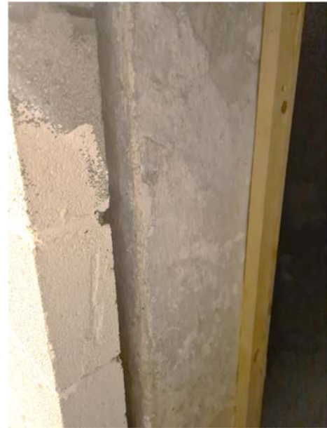
Stone Wall and block build up
