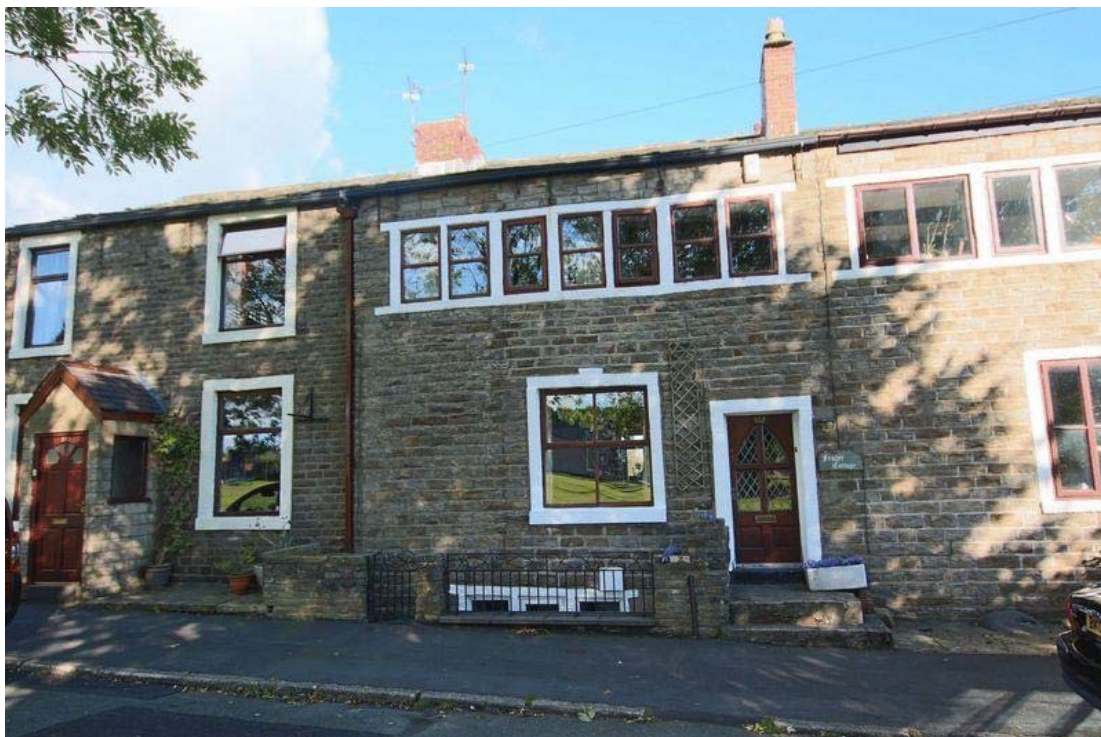
View of the Front (West) Elevation
