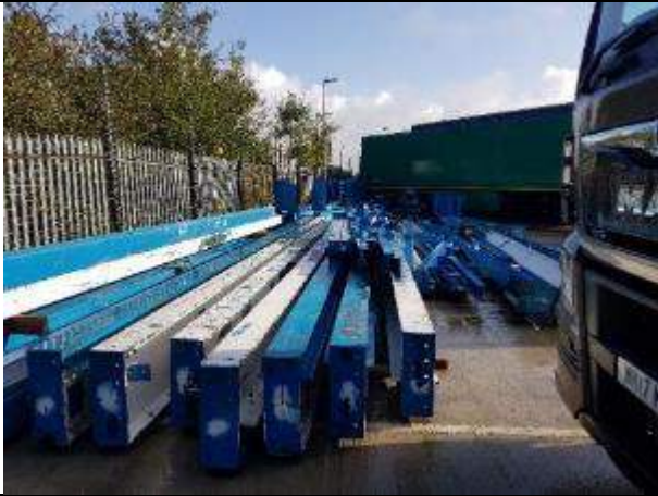
P7: Steel beams located on the northern site periphery
