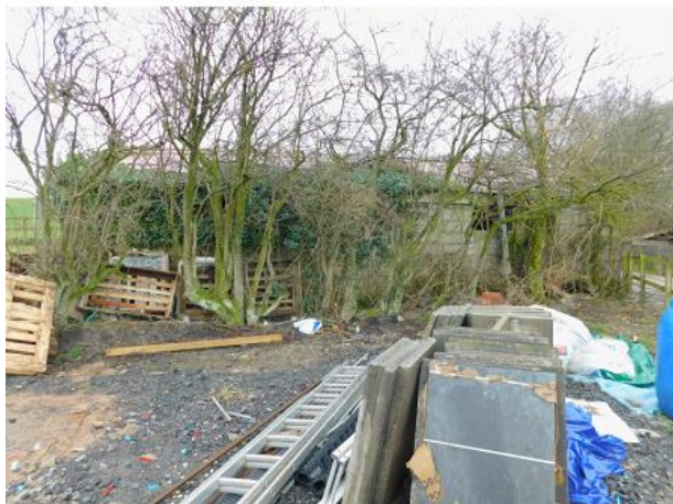
PHOTO 5 Southern Elevation of Chicken Shack
