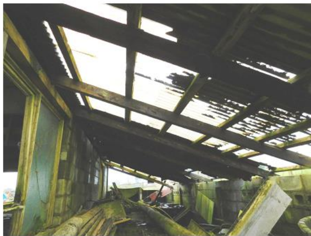
PHOTO 15 Underside of Lean-to Roof
