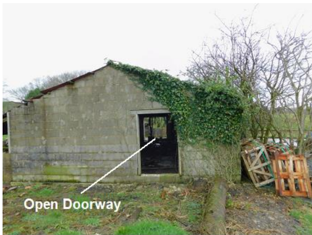
PHOTO 7 Western Elevation of Main Building
