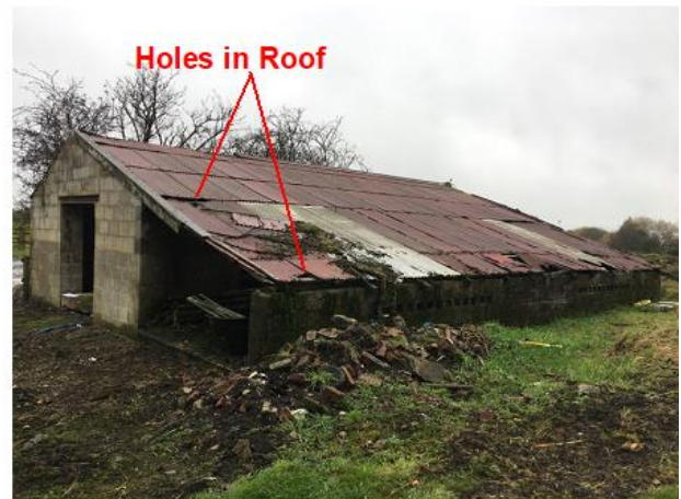
PHOTO 12 North-eastern Corner of Chicken Shack
