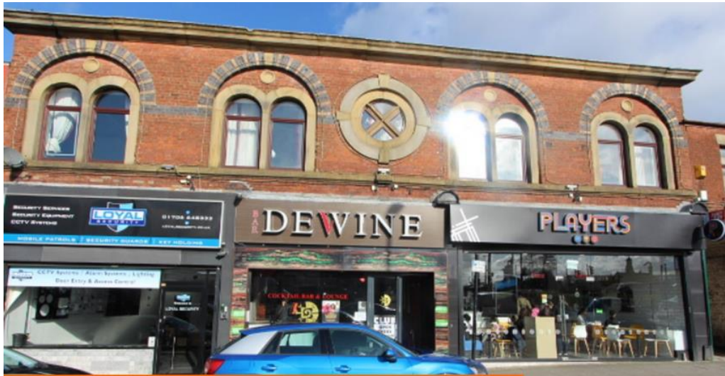
Photo above shows the shopfront as existing.
