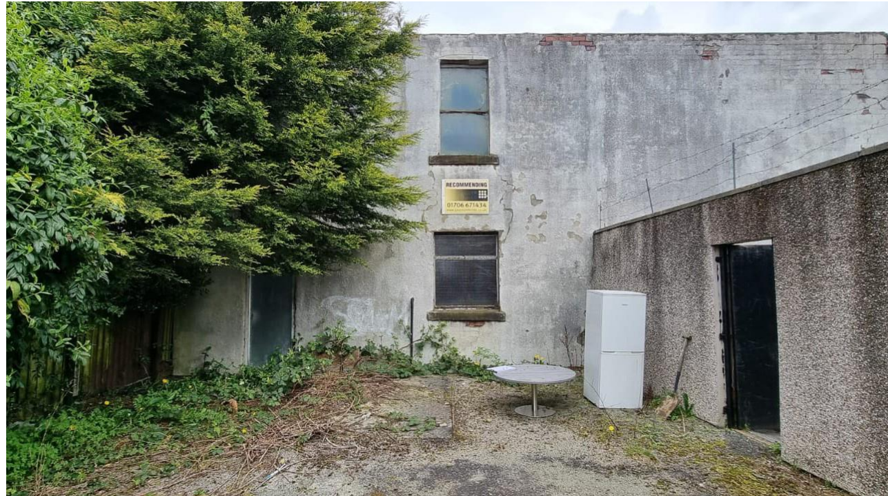
Existing site and building photos. The wall to the right would be removed to create a larger courtyard. Leylandii are outside of site boundary
