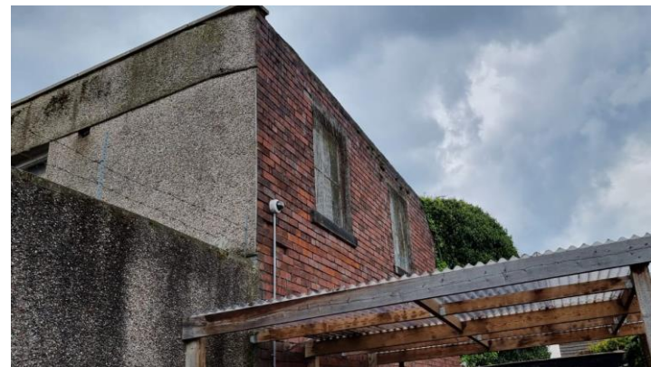
Existing building photos
