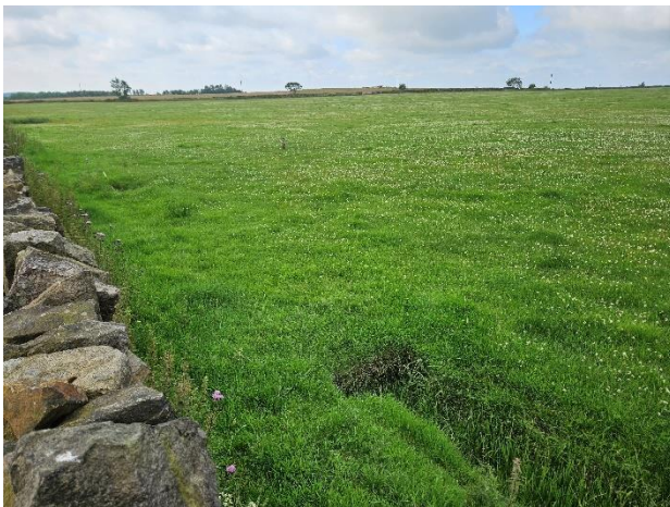
Figure 2.5: Several linear depressions/ collapsed ground parallel to the eastern boundary, along a potential service route.
