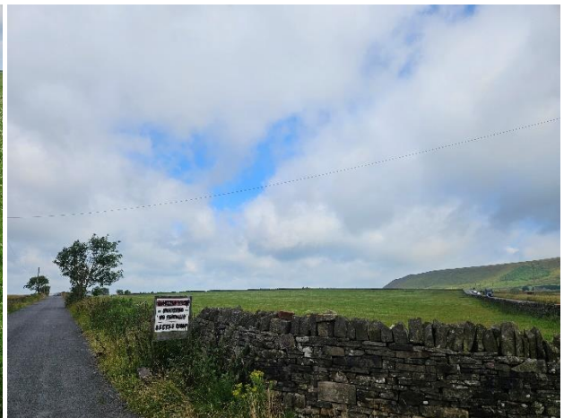
Figure 2.6: Overhead cables crossing the southern section of the site
