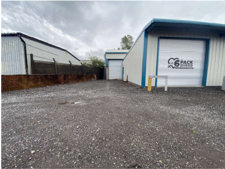
Looking Southeast on Northwest of Business Park
