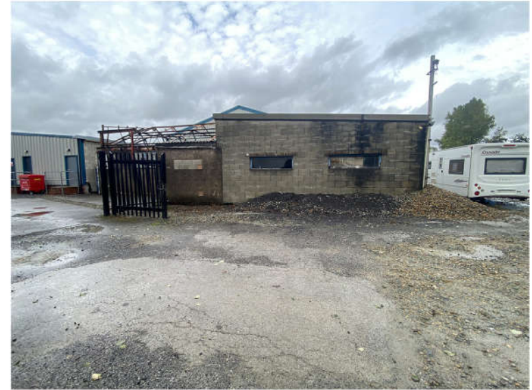
Looking Northeast at Unit 3
