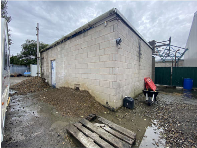
Looking West at Unit 3
