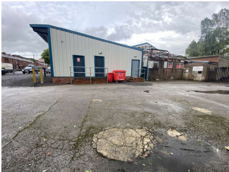
Looking Northeast at Unit 5
