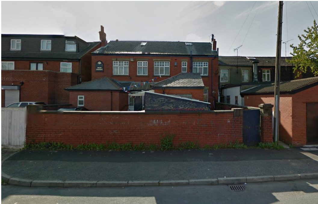
Above: Photo above shows the vehicular entrance into the site from Athol Street and the buildings rear elevation with single storey extensions.
