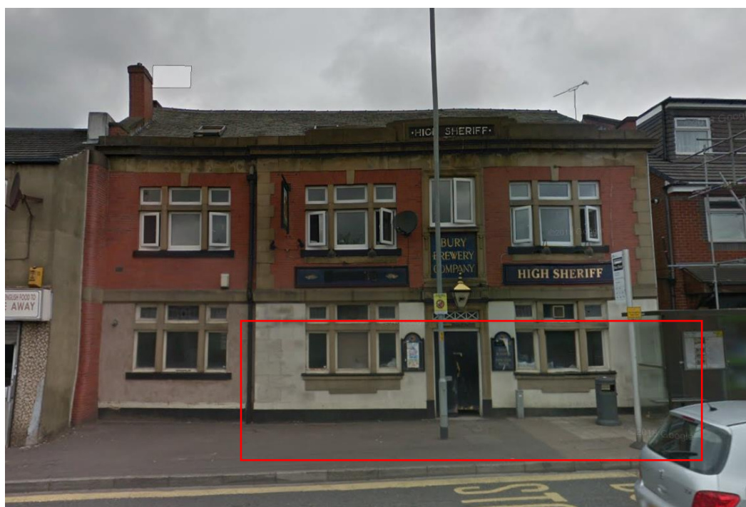
Above: Photo above shows the front elevation of the building and the area to be converted to residential use.
