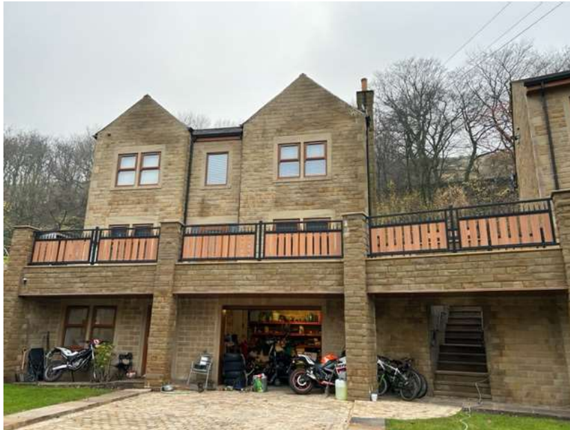
Image 3 – Three storey build at Carp View
