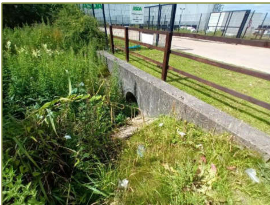
Watercourse 1 channel and highway culvert crossing to the west of the Site.
