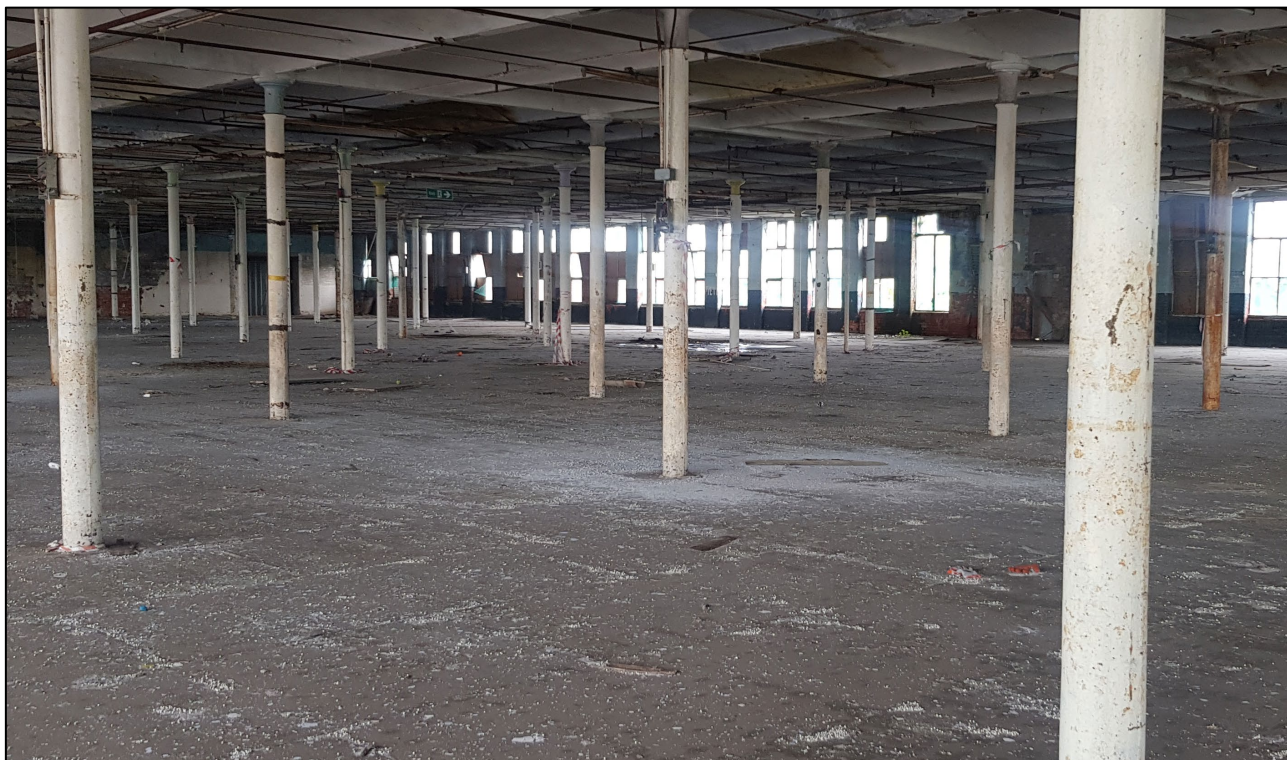
Photo 02. First floor of Warwick Mill (internal survey)
