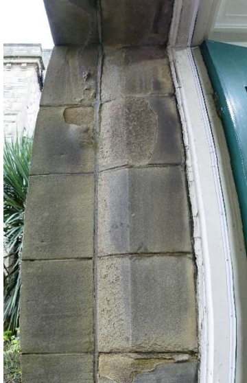
ST1&2- Spalling of face bedded stone around the entrance area. The spalling of the facing to the stone has started at the joints where hard mortar has held water and ice against the outer face of the stone. When this is addressed, a lime mortar should be used to minimise the chance of further spalling.
