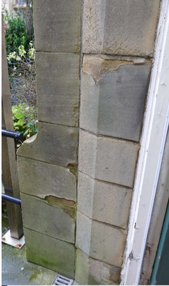
ST1&2- Spalling of face bedded stone around the entrance area. The spalling of the facing to the stone has started at the joints where hard mortar has held water and ice against the outer face of the stone. When this is addressed, a lime mortar should be used to minimise the chance of further spalling.
