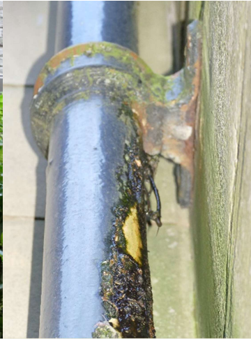
RWP1a&b- The cast iron pipe, to the side of the main entrance, is heavily corroded and leaks, saturating the adjacent wall. Water appears to back up within the pipe and the surface is encrusted with algae and rust.
