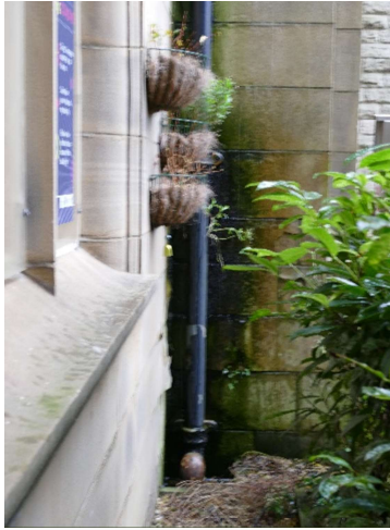
RWP1a&b- The cast iron pipe, to the side of the main entrance, is heavily corroded and leaks, saturating the adjacent wall. Water appears to back up within the pipe and the surface is encrusted with algae and rust.
