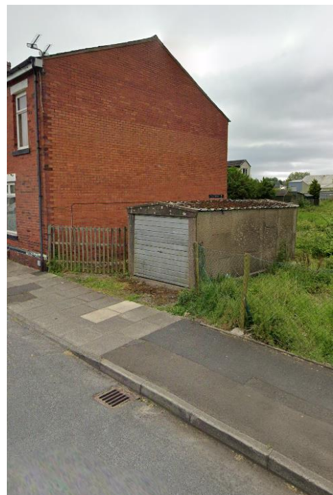
Existing Starkey Street Garage
