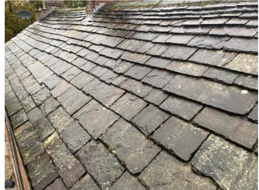
Western elevation of B1a (pictured above).
