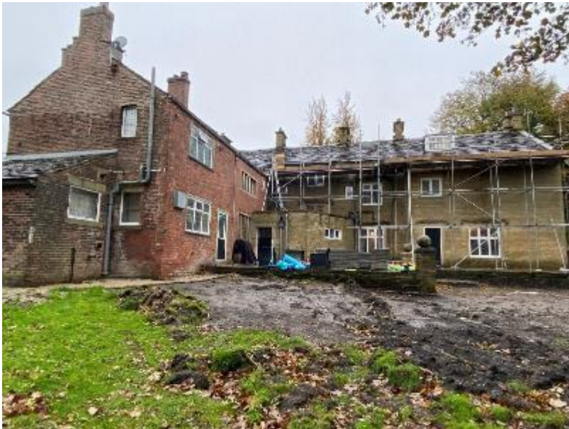
Northern elevation of B1 (pictured above).
