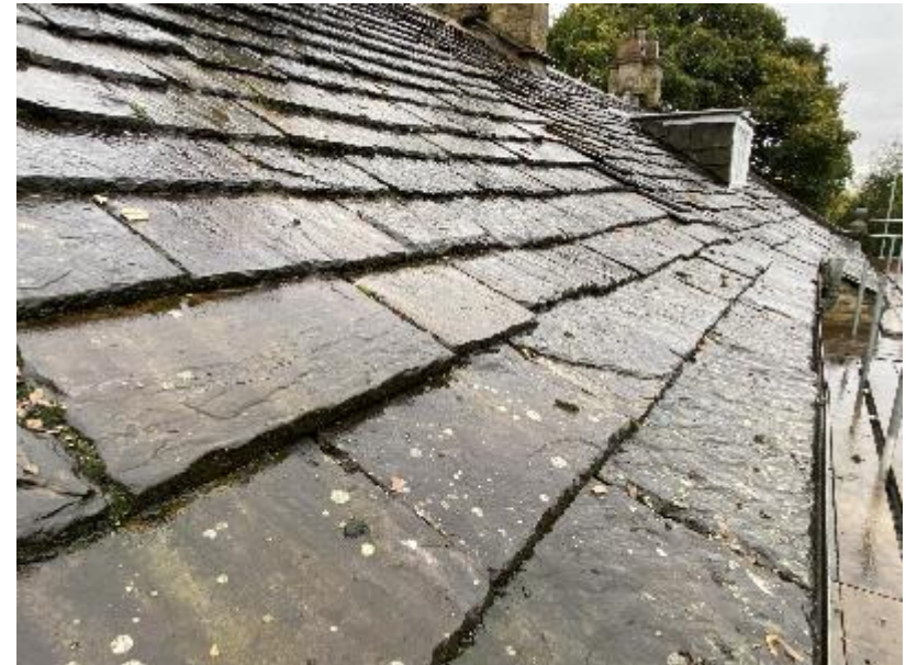
Northern elevation of B1 (pictured above).
