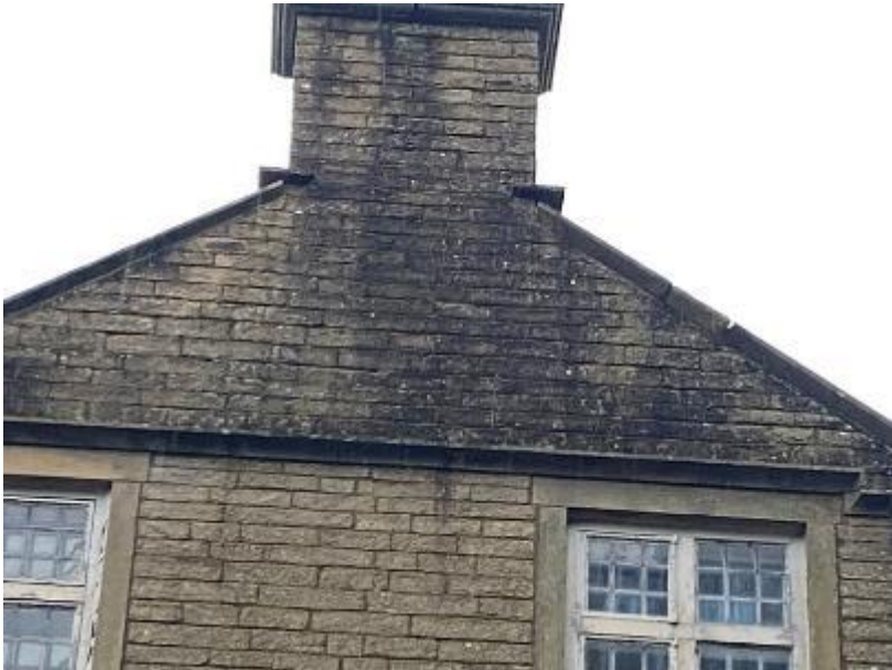
Western elevation of B1 (pictured above).
