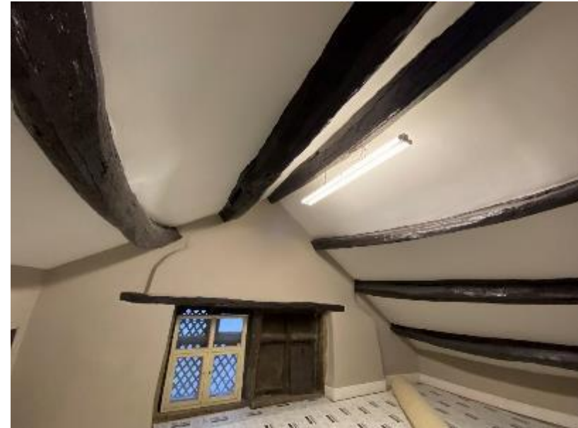
Interior of roof void of B1 (pictured above).
