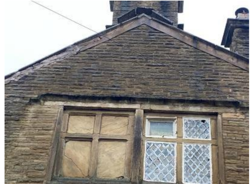
Eastern elevation of B1 (pictured above).
