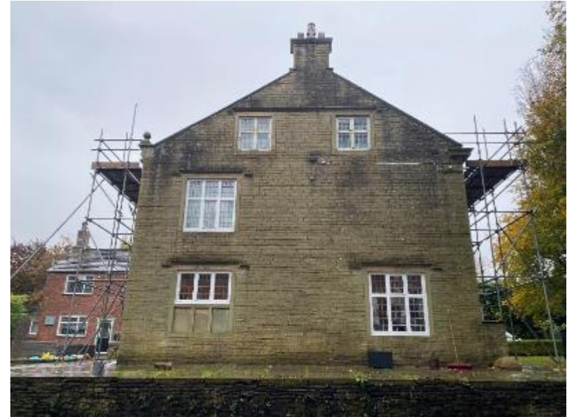
Western elevation of B1 (pictured above).
