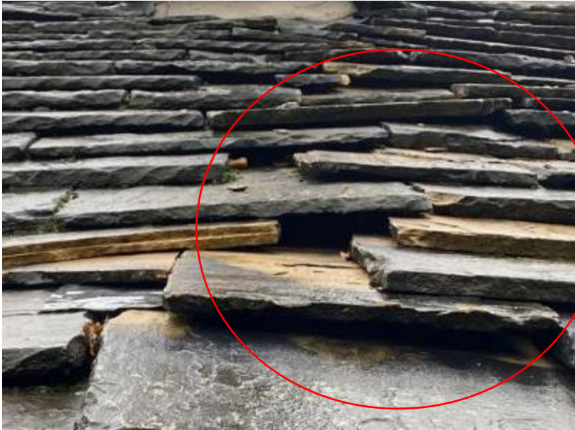
Northern elevation of B1 (pictured above).
