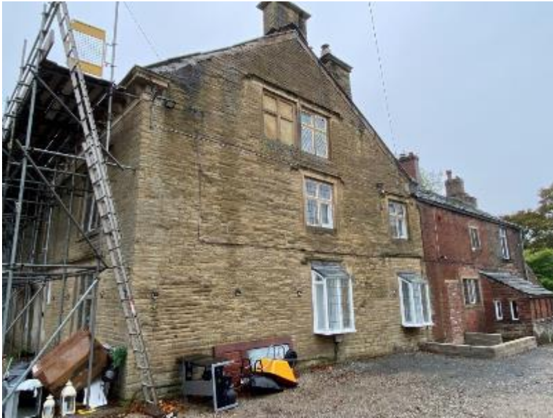
Eastern elevation of B1 (pictured above).
