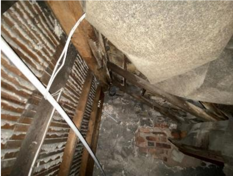
Crawl space within roof void of B1 (pictured above).
