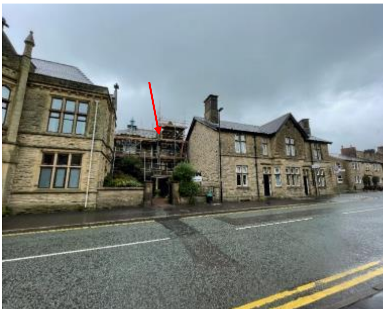
Plate 35: The Milnrow Carnegie Library (red) as seen from Newhey Road, set amongst the town hall and police station.
