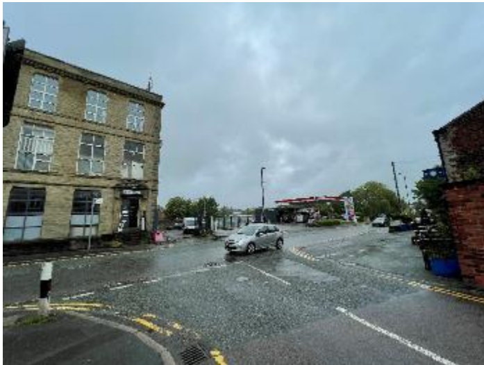
Plate 4: Albert Mill as seen from the east alongside the petrol station located to the north of the Site.
