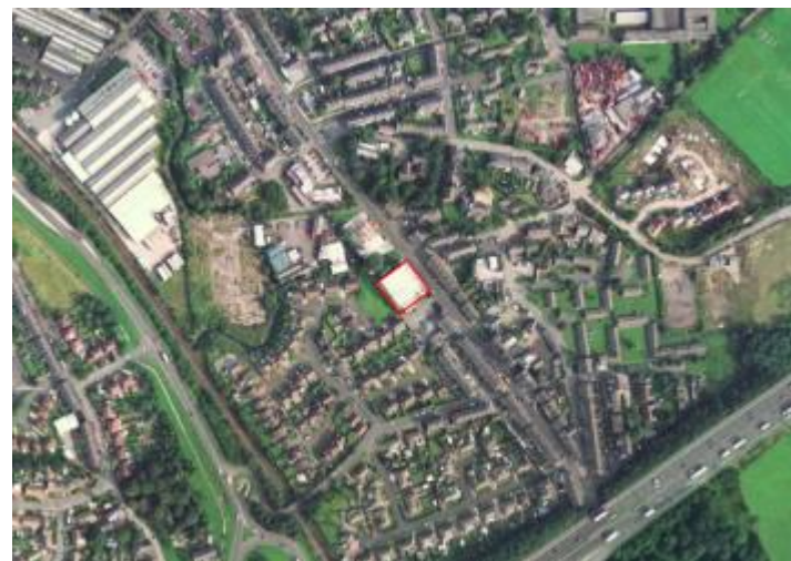
Plate 15: Aerial photograph of the site (red) and its environs, 2000.
