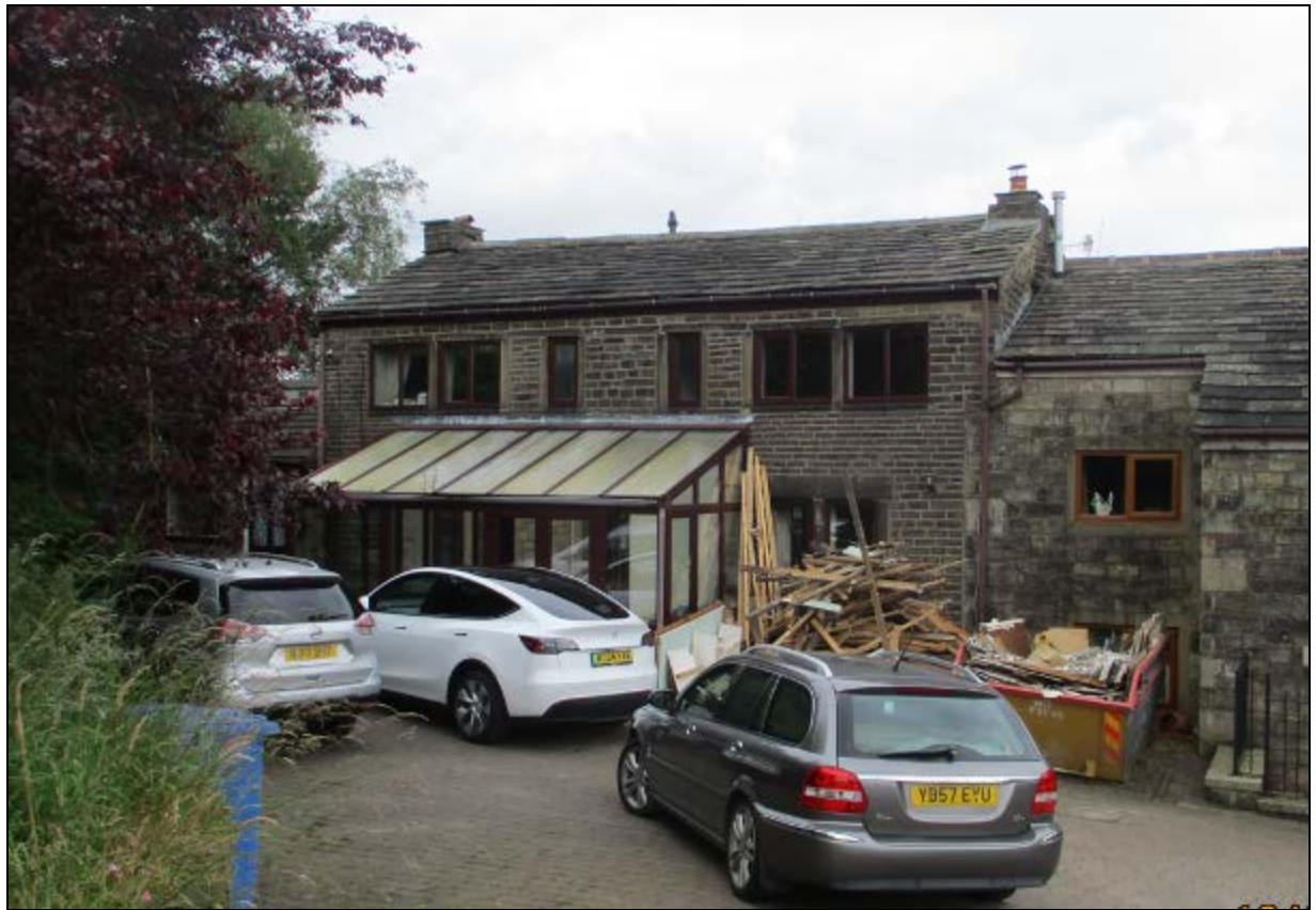
1. The application property, a modest former farmhouse with attached barn
