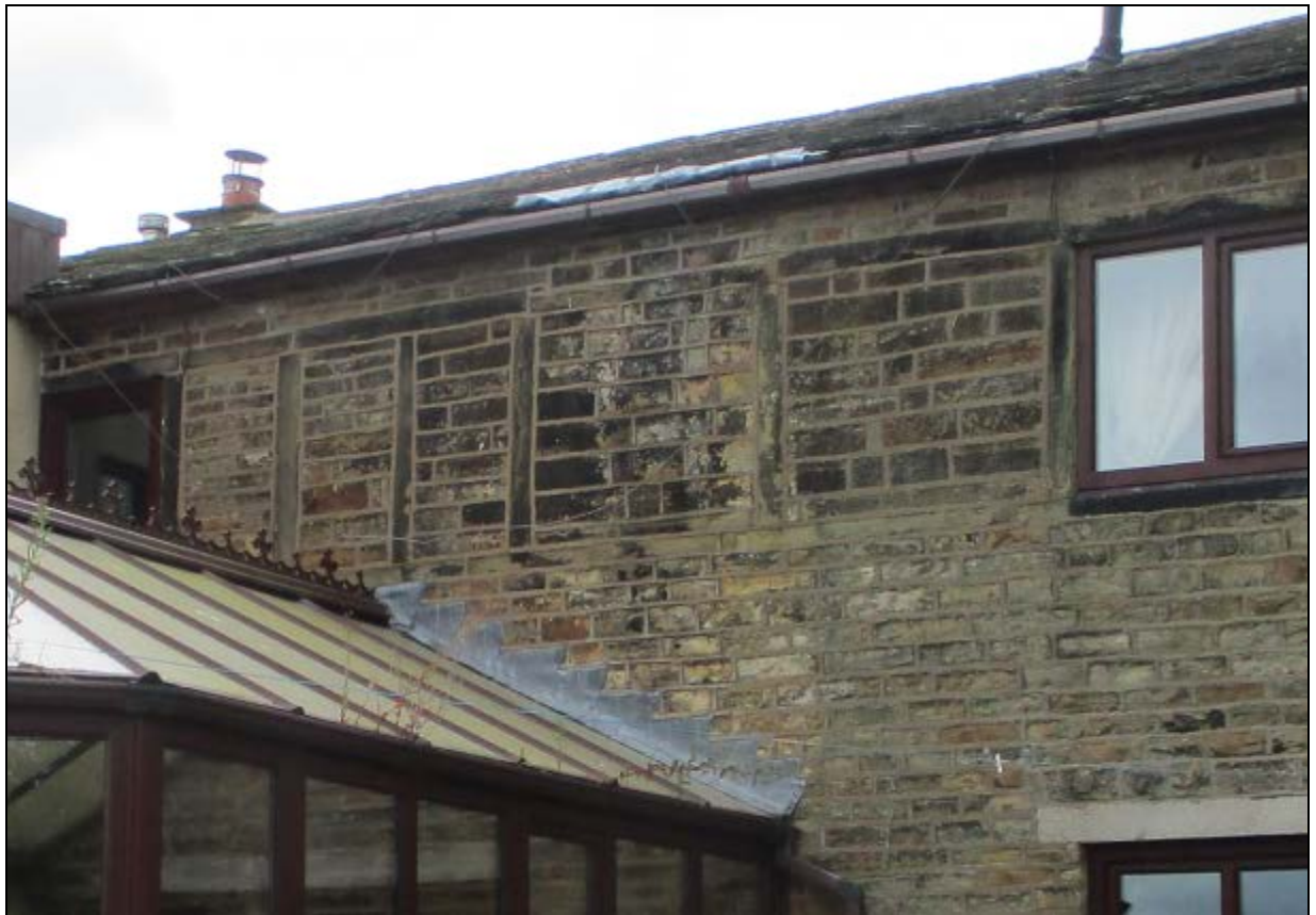
3. Blocked windows indicate first floor loomshops originally existed
