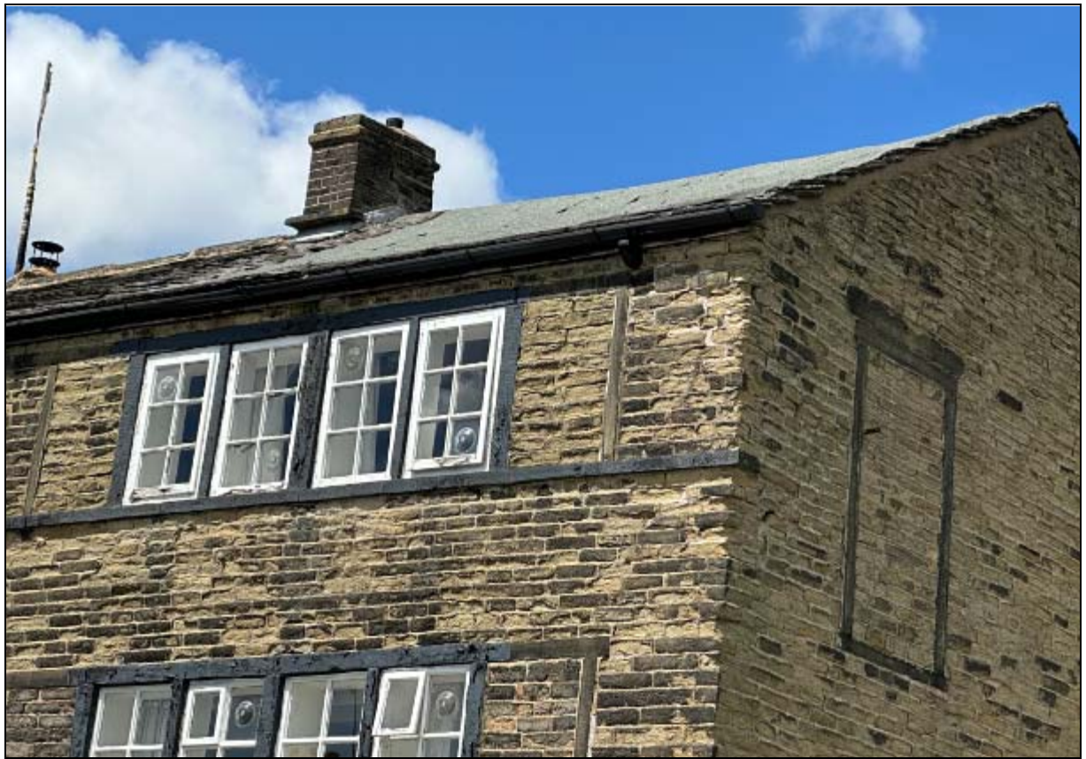
4. Long mullioned windows and blocked taking-in door indicate origins as a weaver's cottage
