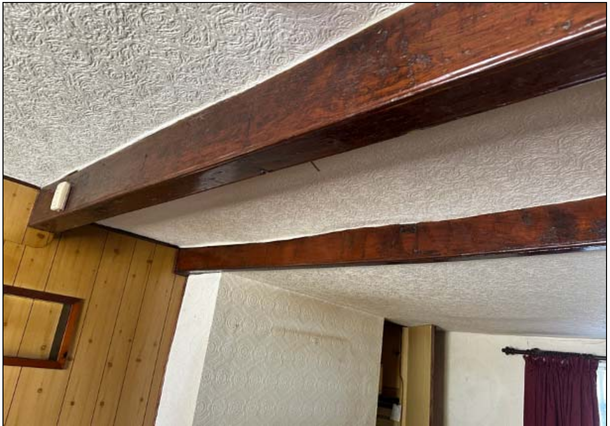
12. Beams and chimneybreasts are the sole surviving historic internal features
