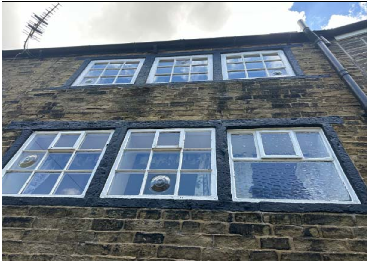
6. Wide mullioned windows on rear elevation
