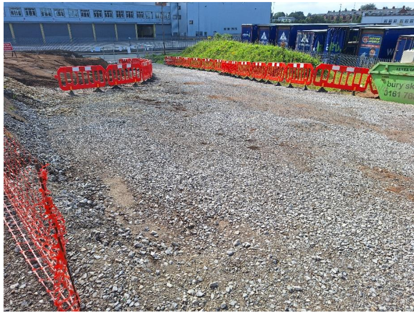
Figure 5 Showing Gravel Access Track
