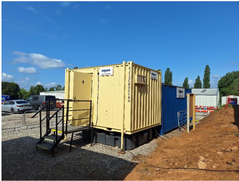
Figure 7 Showing Welfare Units
