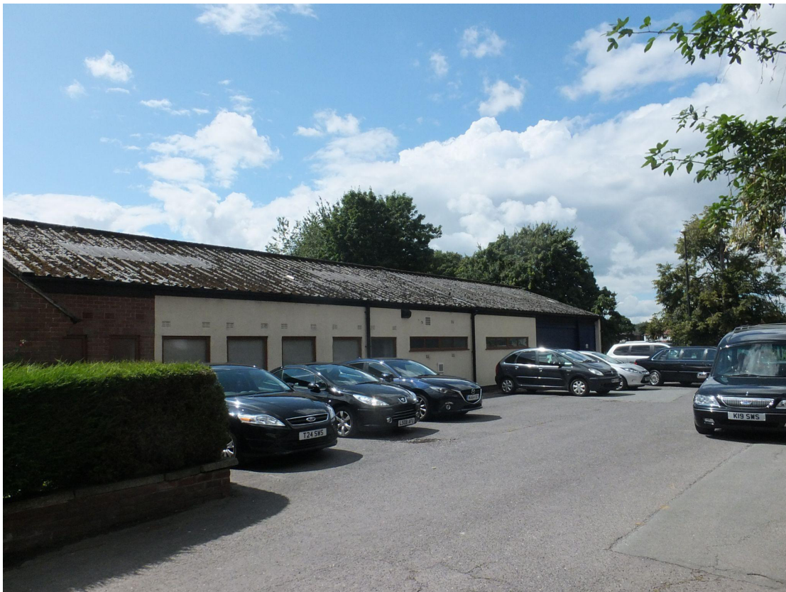
Rear Northern wing, showing existing asbestos roofing panels.
