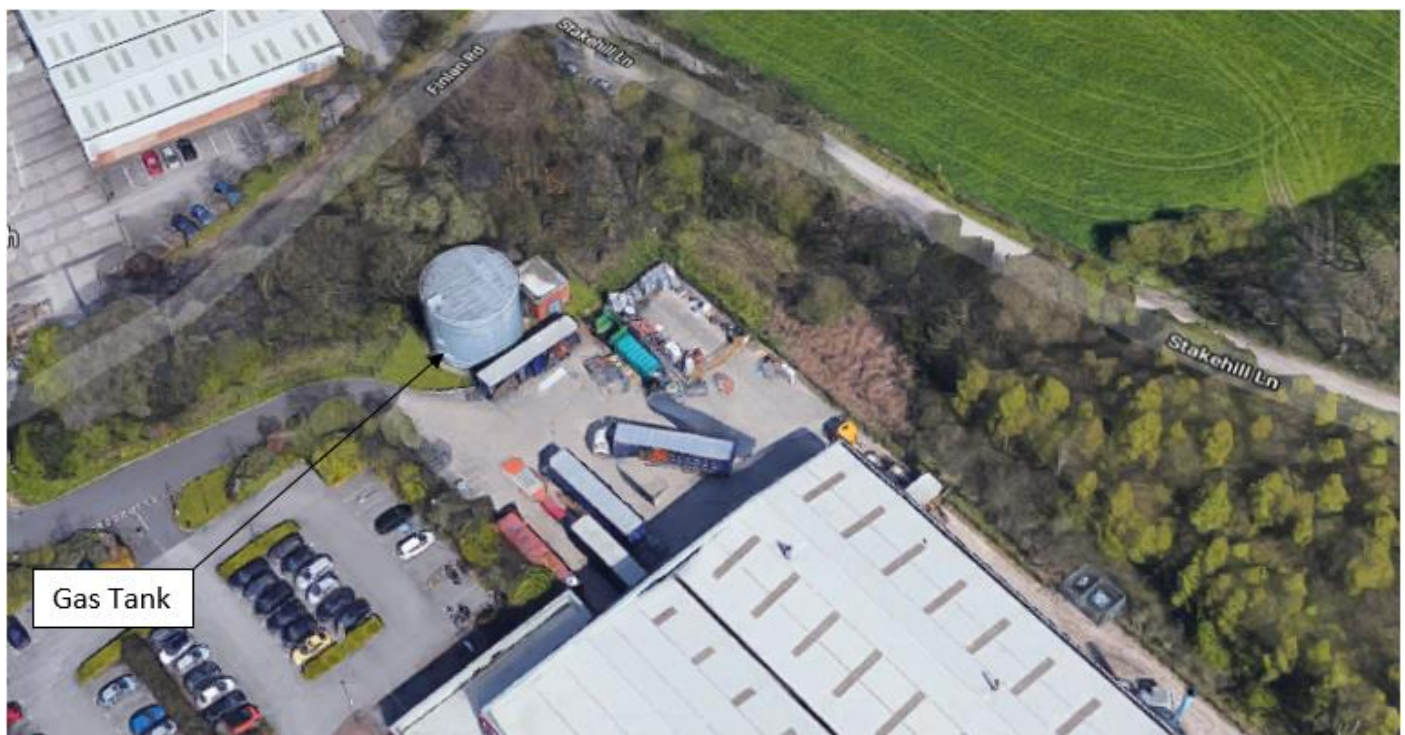
Figure 8.1 – Medium Pressure Gas Storage Tank
