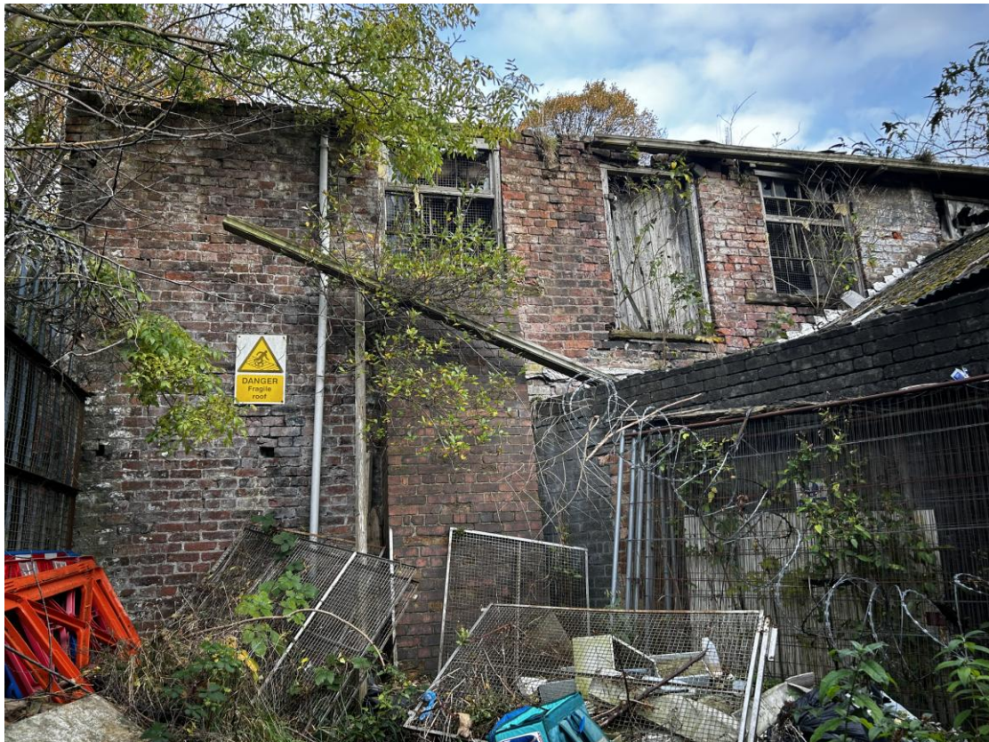
Current condition of building
