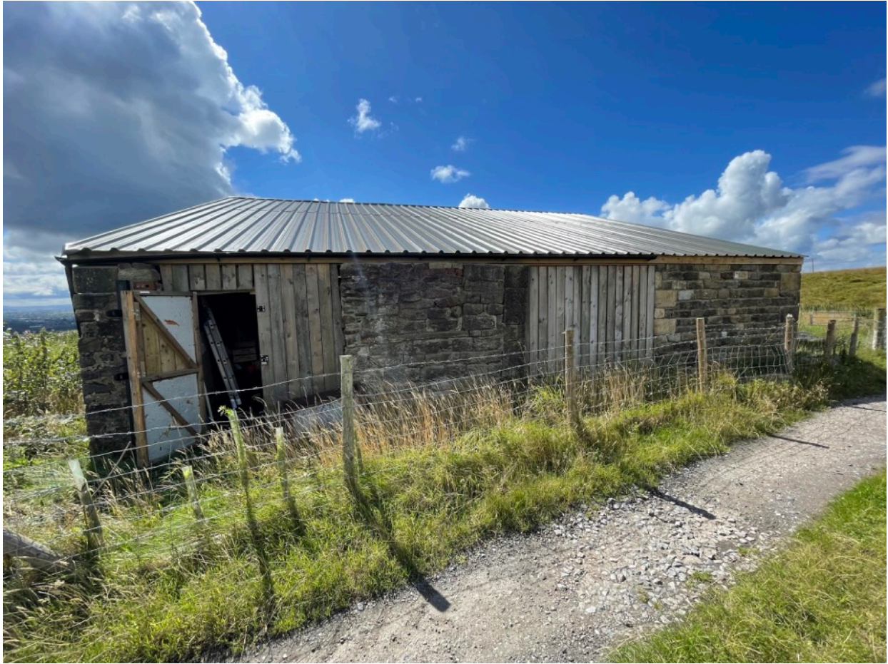
Exterior of the barn- North elevation facing Fordoe Lane
